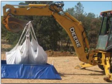
Figure 12. Extracting the concrete solids or gelled washwater
