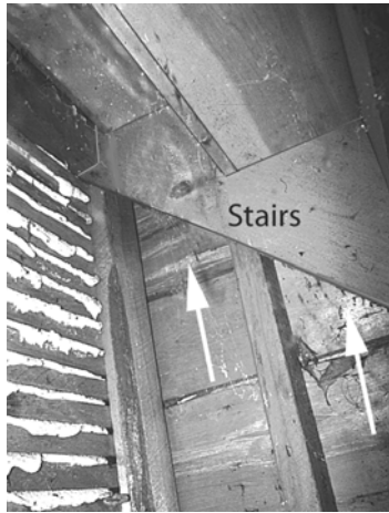
Insulating and sealing attic stair walls, doors, and stairs: Insulating and air sealing these is one way of establishing the thermal boundary.
