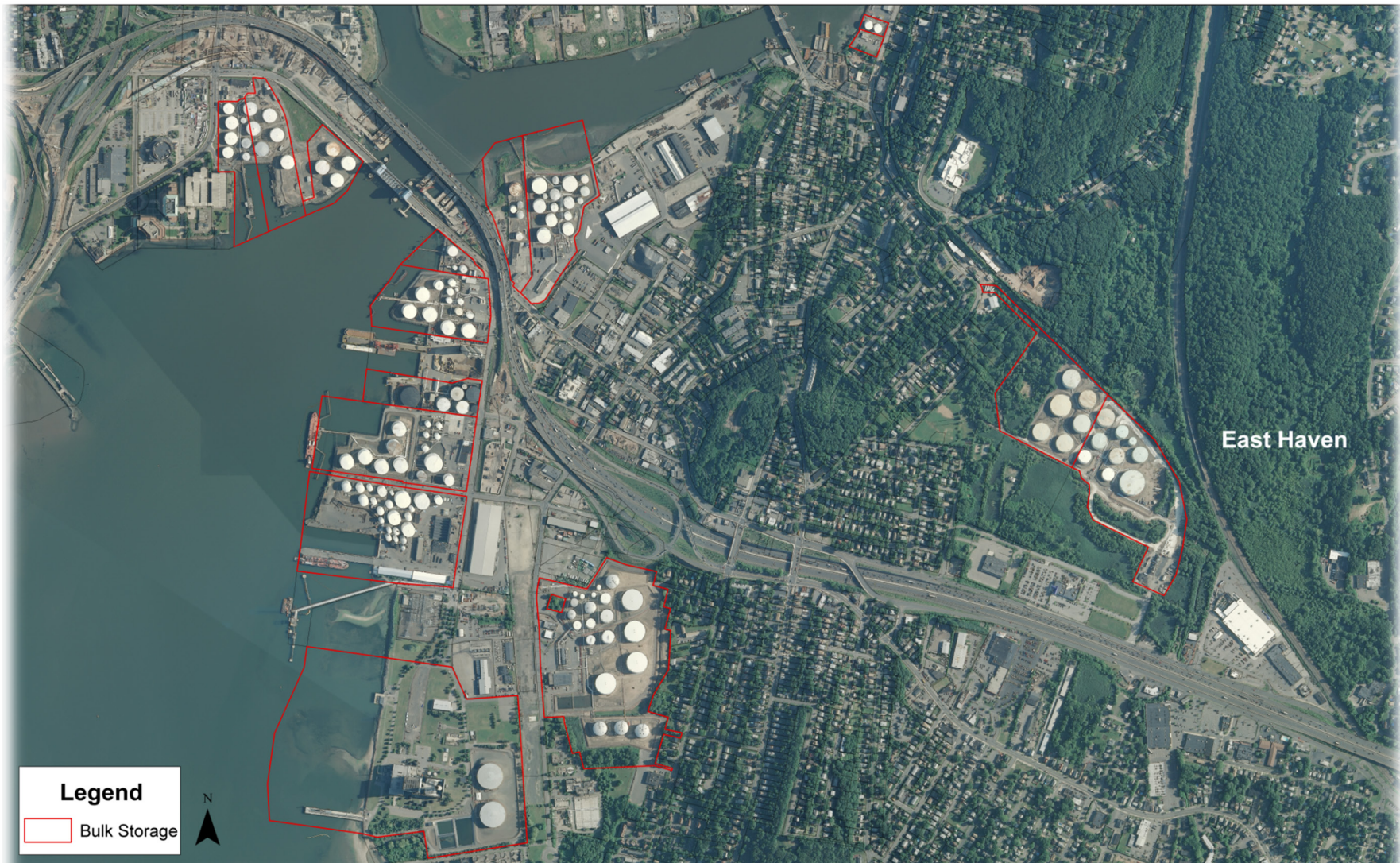
Figure 7: Port of New Haven Parcels Containing Bulk Storage: Total Acres 254.88
