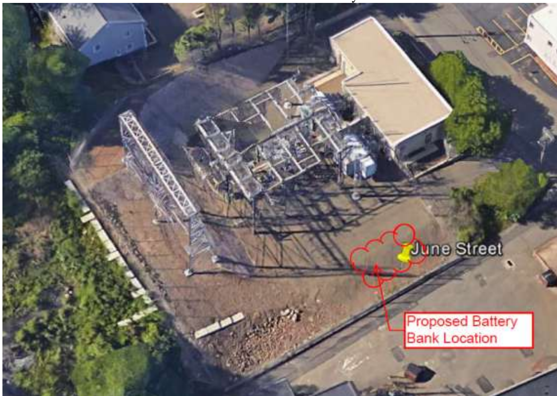
June Street Substation (4 Hazel Terrace, Woodbridge, CT) Google Earth 2017
