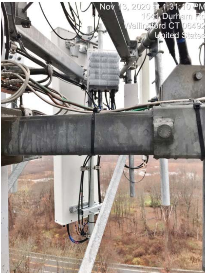
Gamma Sector: (1) New Antenna & (1) New RRH Mounted To The Reinforce Mounting Platform On The Existing Monopole
