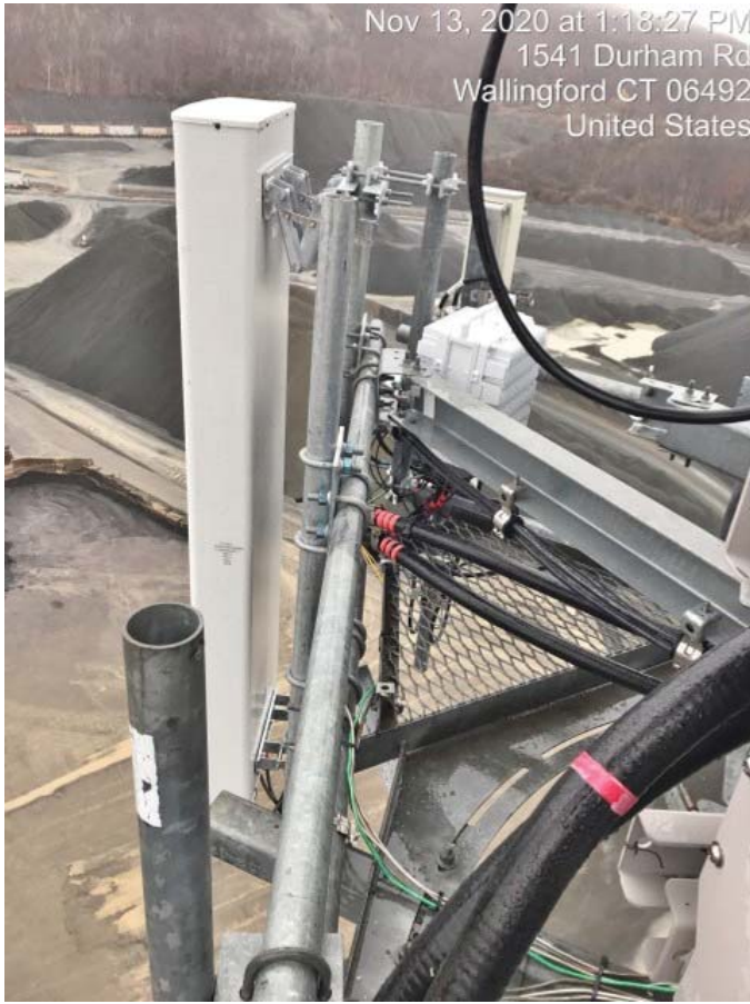
Alpha Sector: (1) New Antenna & (1) New RRH Mounted To The Reinforce Mounting Platform On The Existing Monopole
