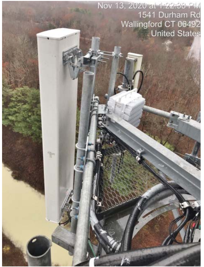
Beta Sector: (1) New Antenna & (1) New RRH Mounted To The Reinforce Mounting Platform On The Existing Monopole
