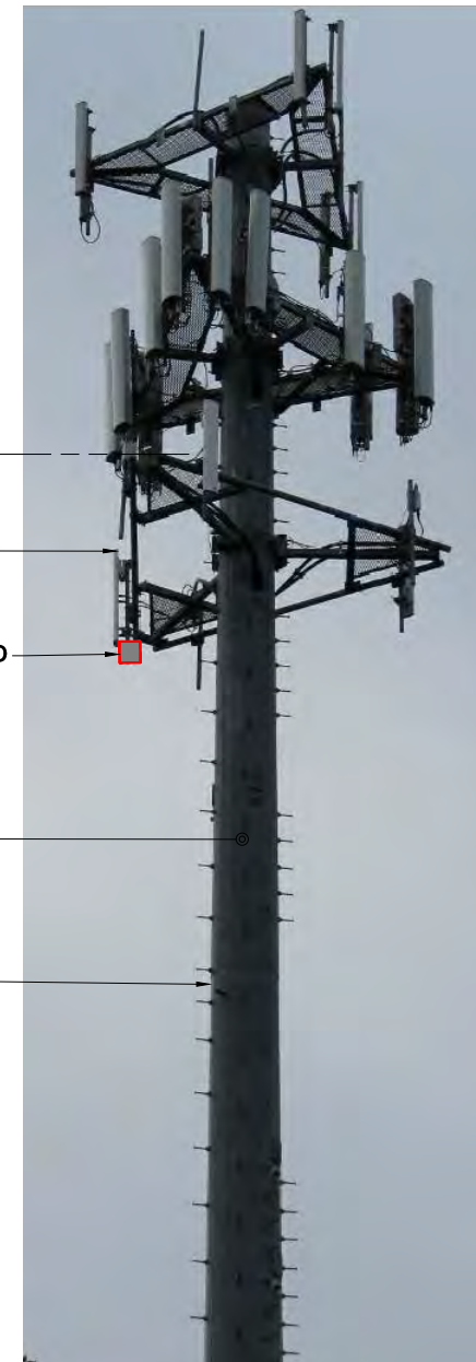
ELEVATION PHOTO DETAIL N.T.S.
