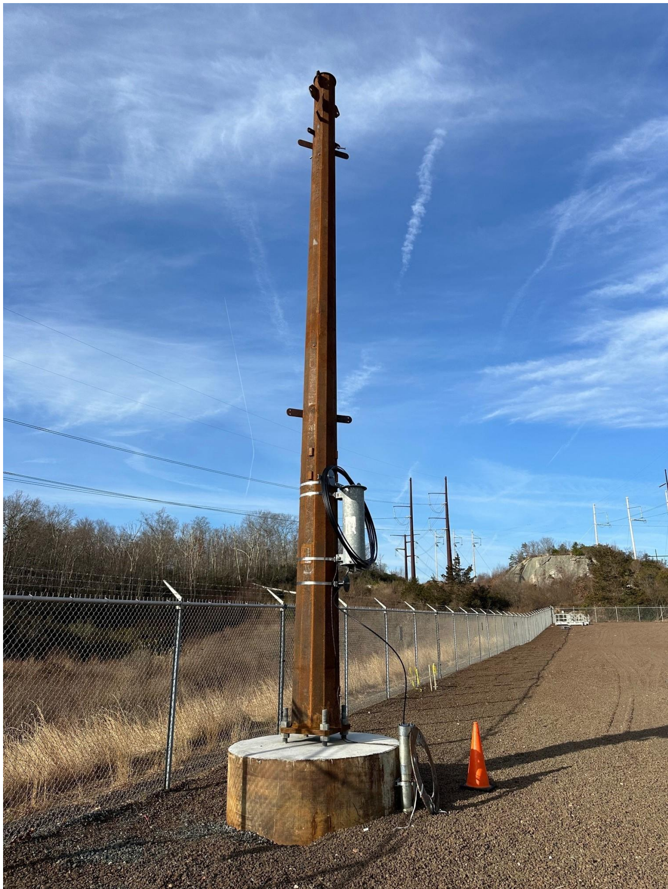
Attachment A: Photograph of Stub Pole: Scovill Rock Switching Station
