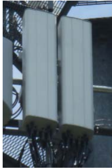
Dual mount panel antennas
