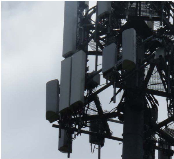
Verizon Sector with new radios
