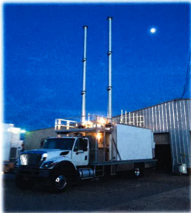
Temporary Telecommunications Facility 156 Sterling City Road Lyme, CT
