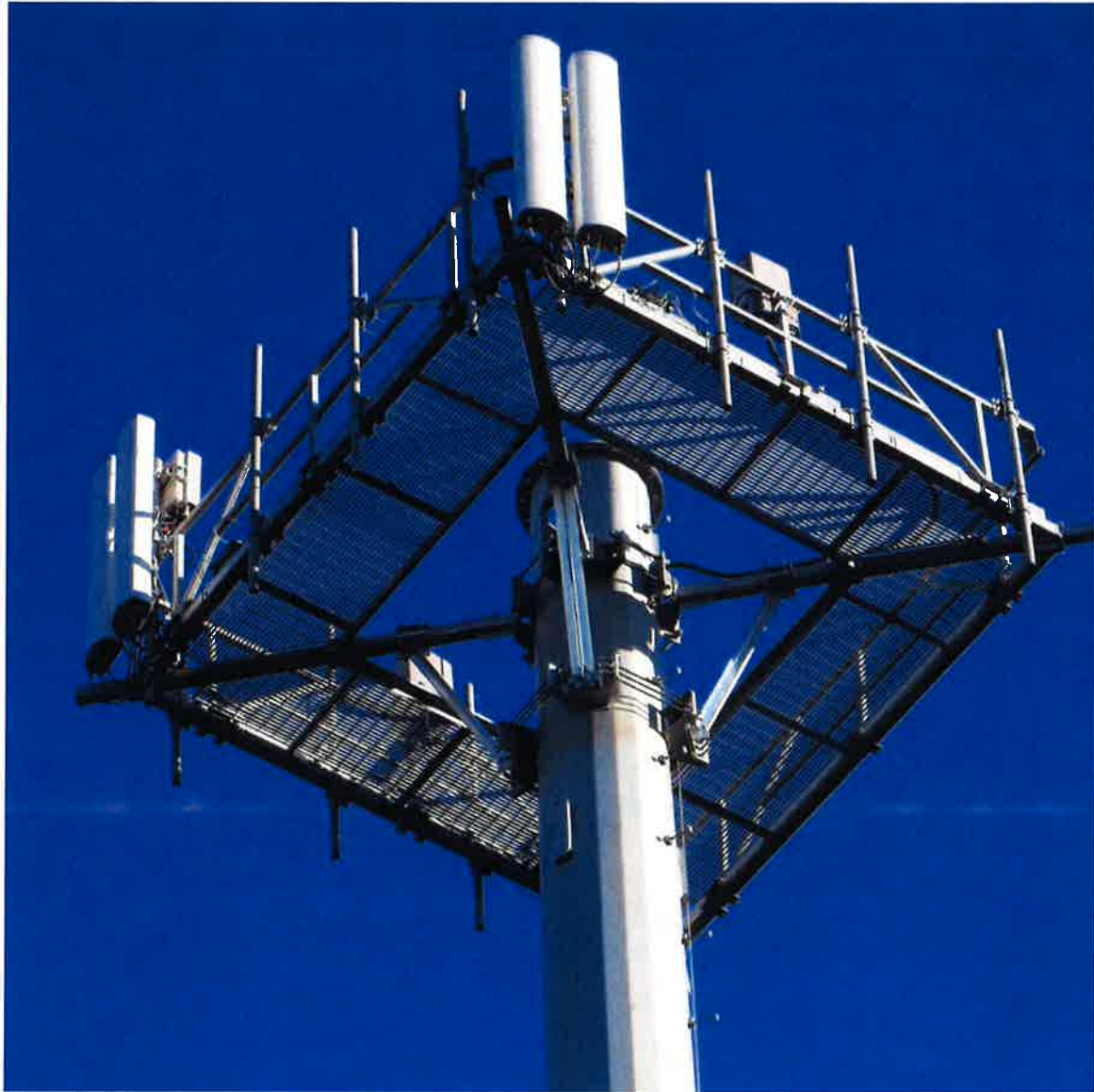
Photo 1: Photo illustrating the Monopole with Appurtenances shown.
