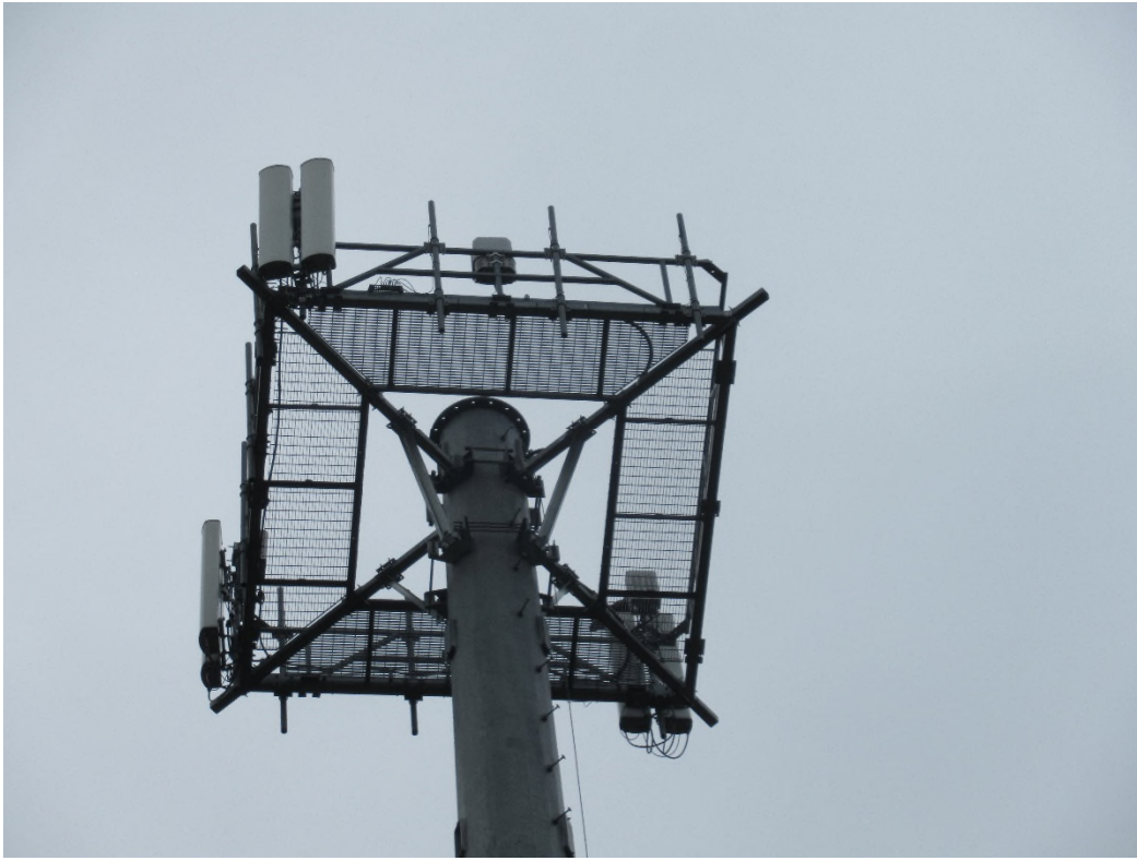
Photo 1: Photo illustrating the Monopole with Appurtenances shown.
