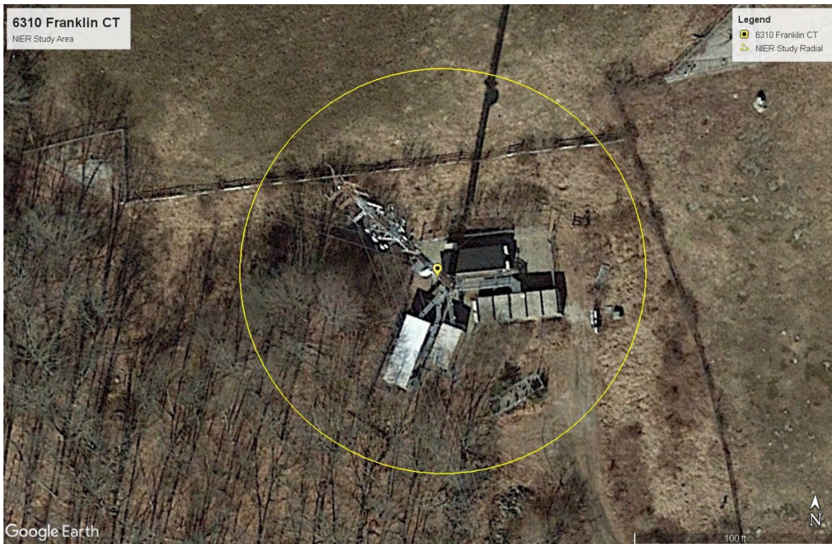
Aerial View of Site
