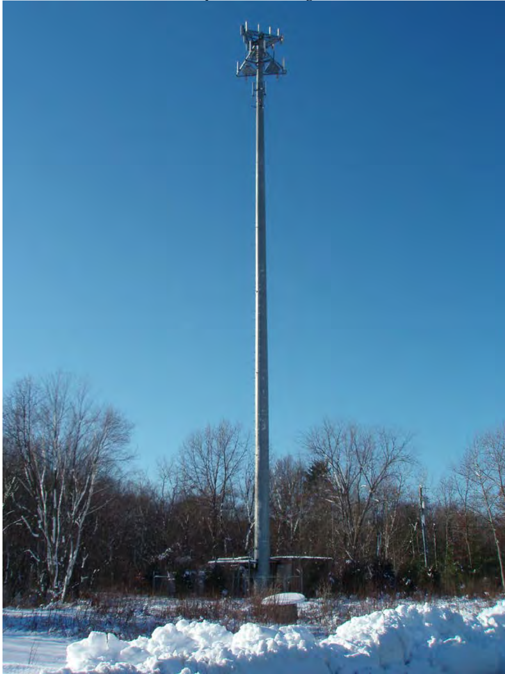
Close up view of existing tower
