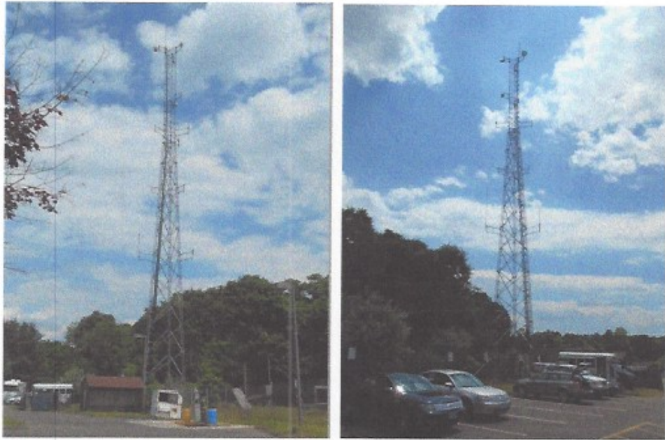
Overview photos of 160' self-supporting tower.
