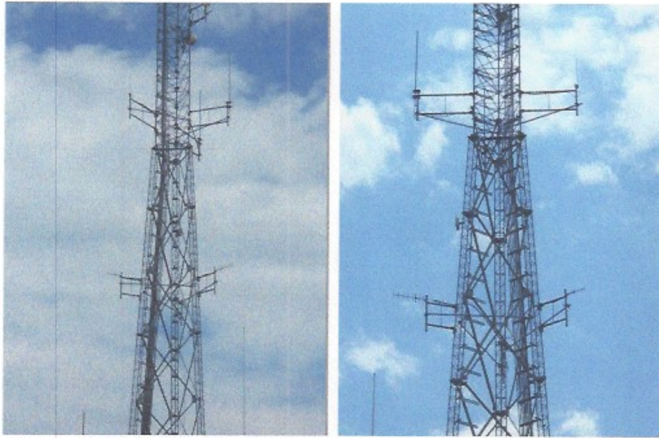
Photos of mid-section of tower, showing existing equipment.
