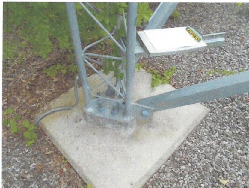
Photo of typical foundation pier.
