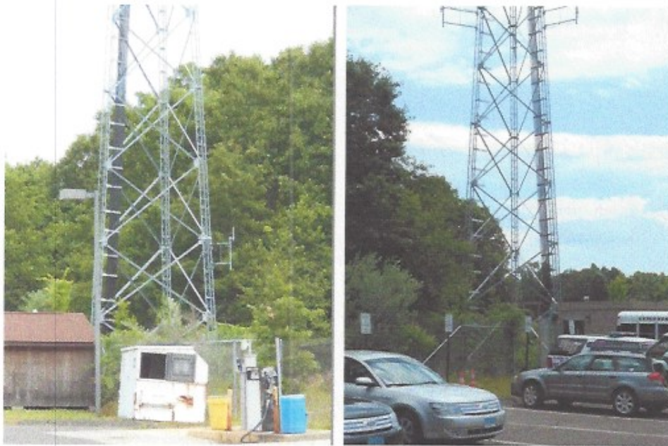
Photos of bottom of tower.
