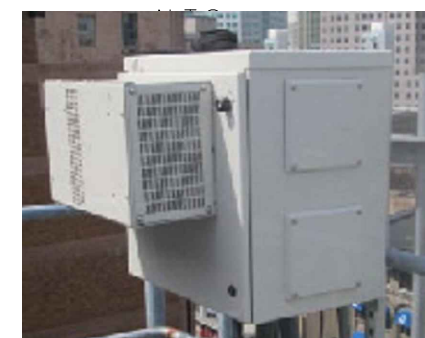
EMERSON NETXTEND COMPACT 2416 CABINET ENCLOSURE: ALUMINUM DIMENSIONS (HxWxD): 24" X 24" X 25.25" WEIGHT: 64LBS (EXCLUDES EQUIPMENT) WEATHER TIGHTNESS: NEMA TYPE 3R
