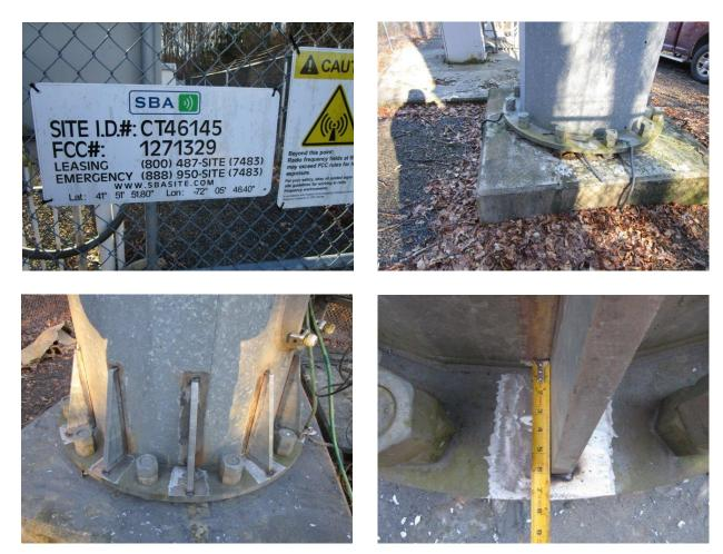
Installation of new stiffeners at the base plate. Deviations: None. Comments: No deficiencies found.
