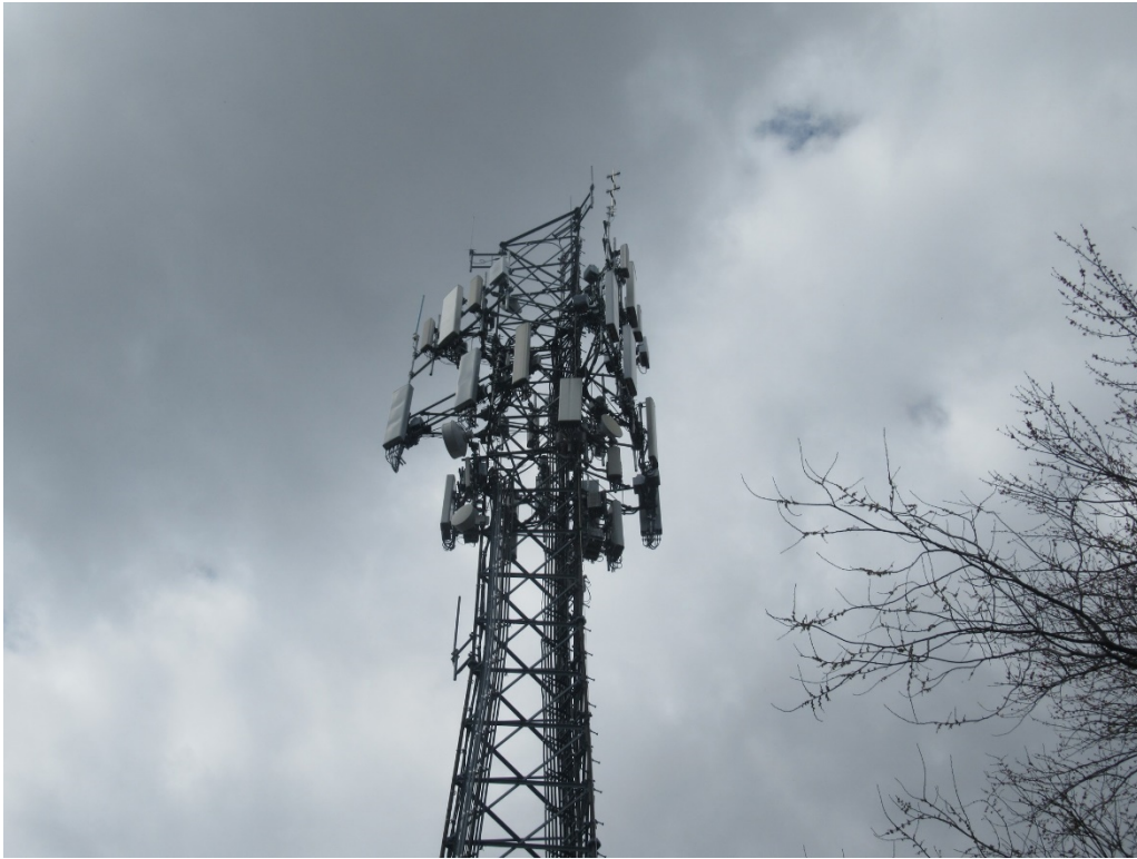
Photo 1: Photo illustrating the Tower with Appurtenances shown.
