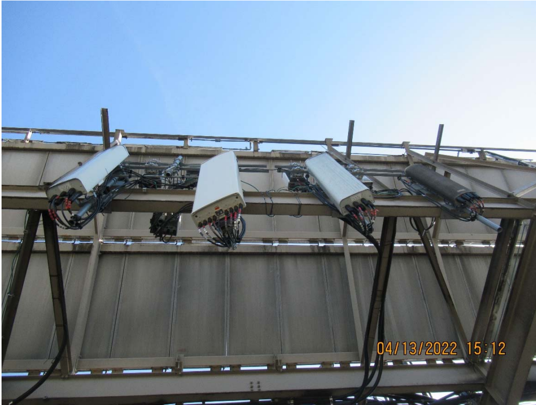
Photo 1: Sample photo illustrating the existing Alpha sector.
