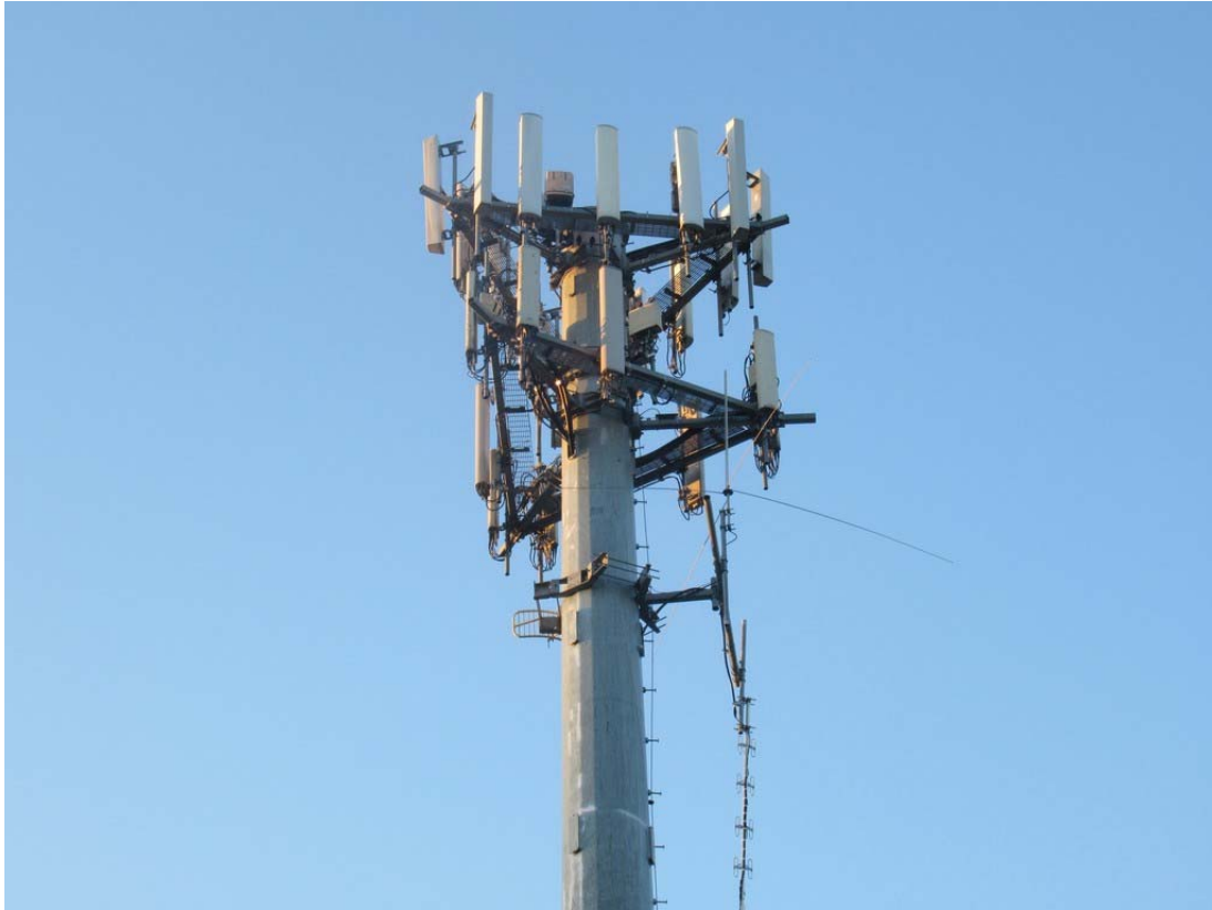
Photo 1: Photo illustrating the monopole with Appurtenances shown.
