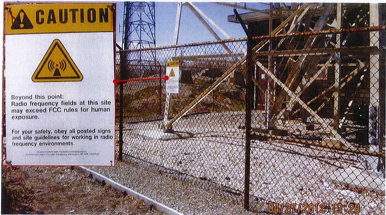
Figure 5: Signage along Southeast Side of Compound
