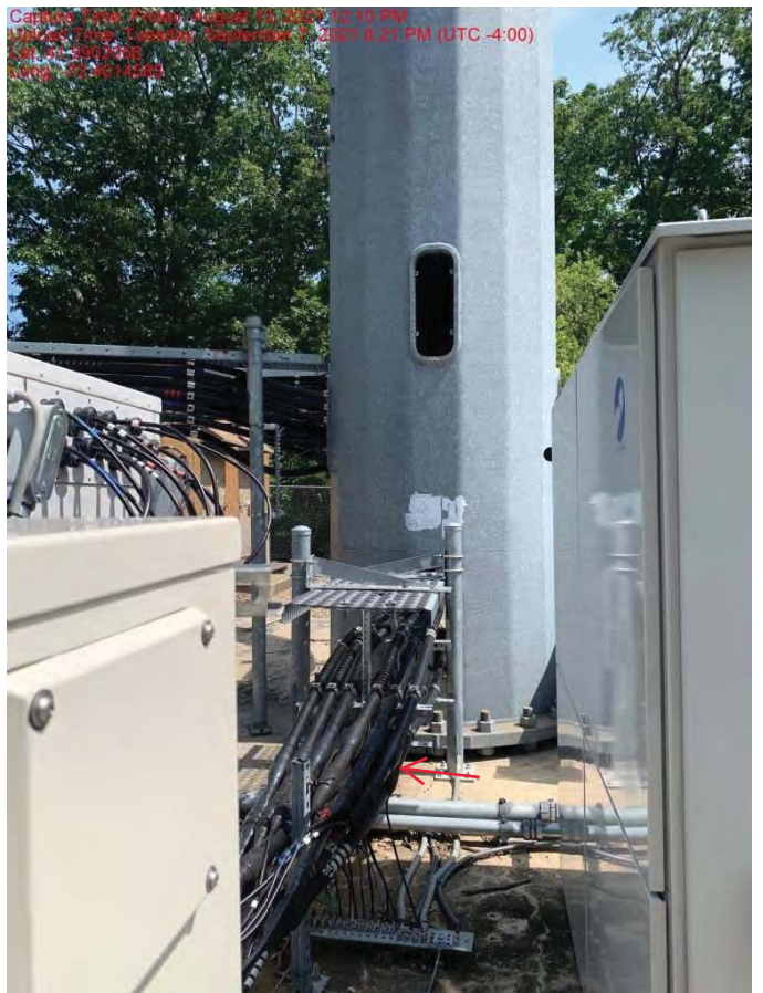
New Signal Cables Run Along Existing Cable Path
