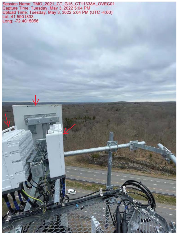
Alpha Sector: (1) New Antenna & (2) New RRHs Mounted To The Modified Platform
