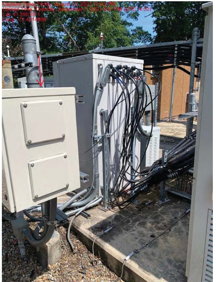
New Purcell Cabinet Installed On Existing H-Frame
