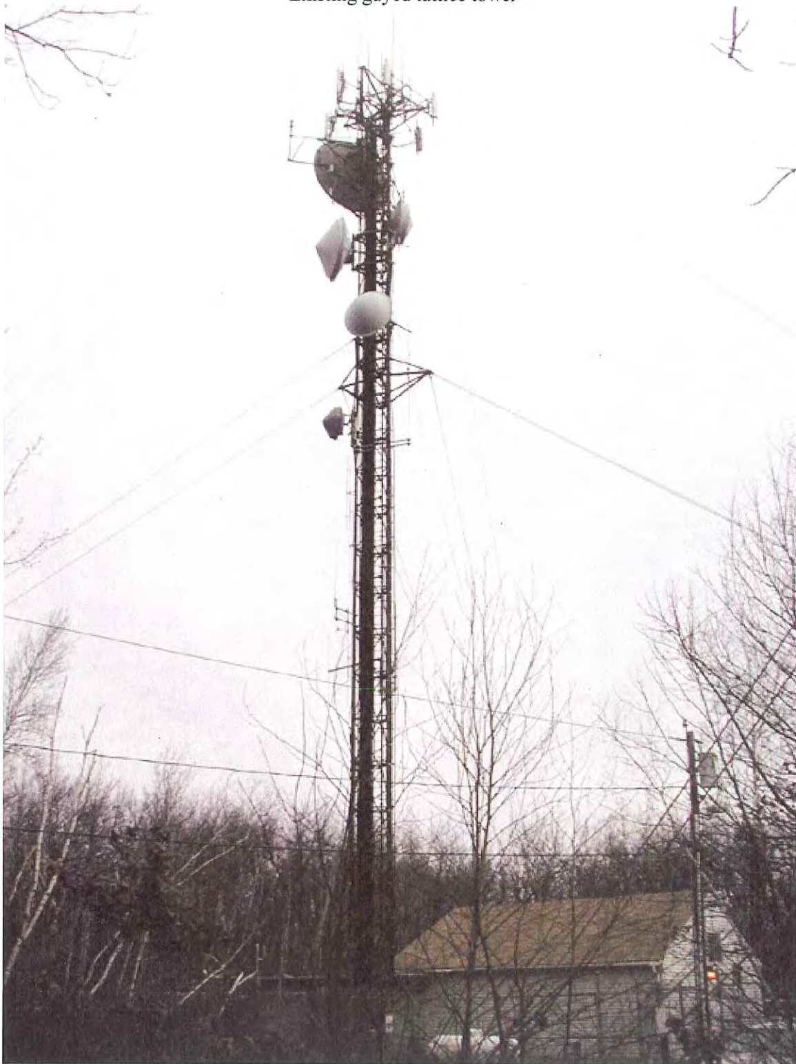
Existing guyed lattice tower
