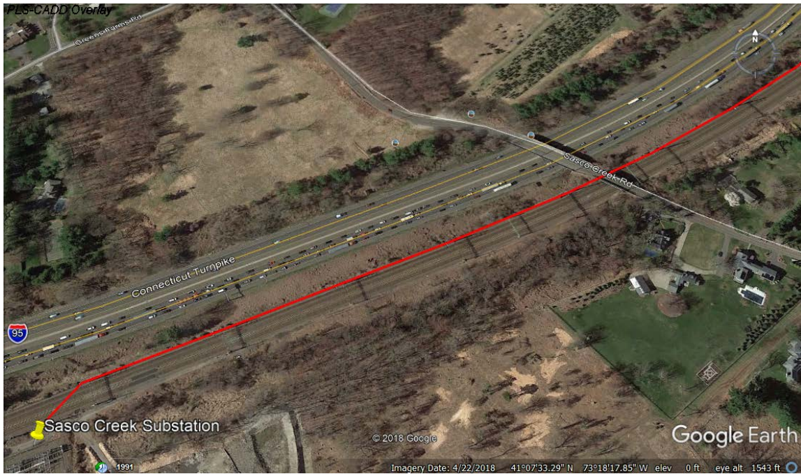
Eversource's Sasco Creek Substation - Google Earth 2/23/19
