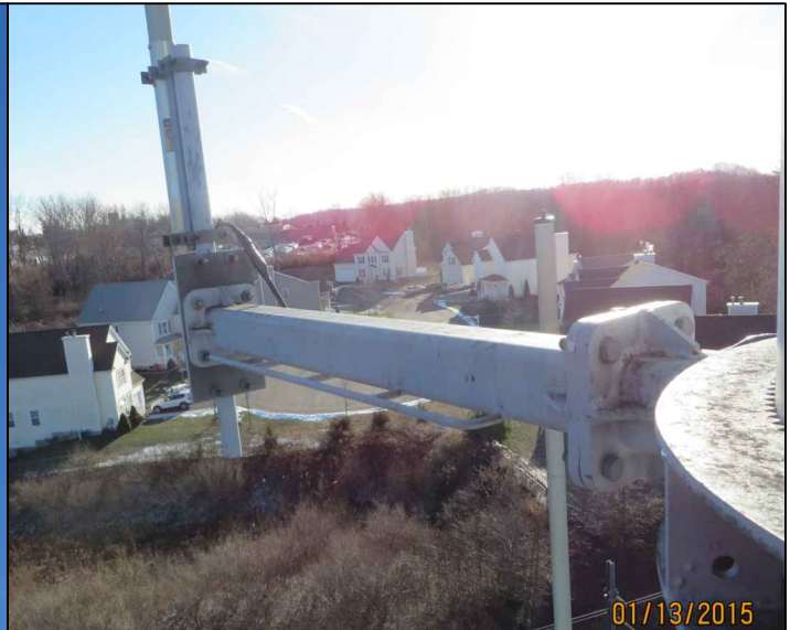
Photo From Tower
