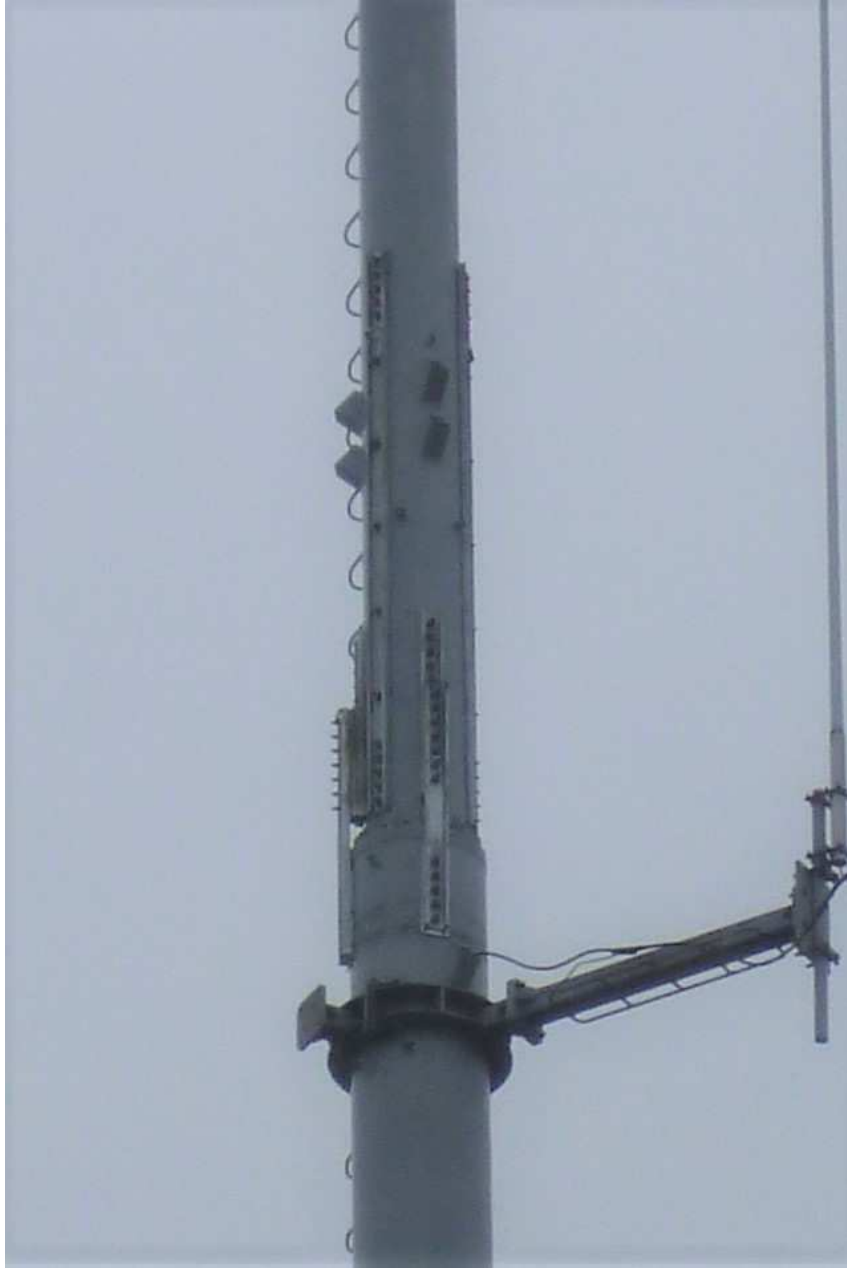
Photo 3: Reinforcement Channel w/Bridge Stiffeners from approximately 99' to 111'
