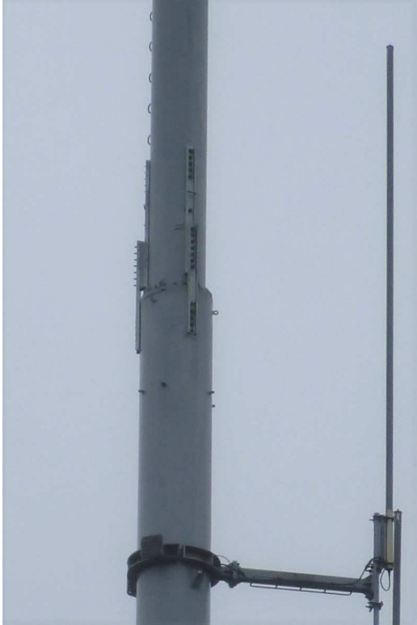
Photo 4: Reinforcement Channel w/Bridge Stiffeners from approximately 79' to 86'
