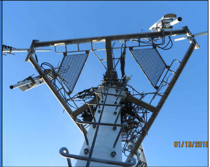
Photo From Tower
