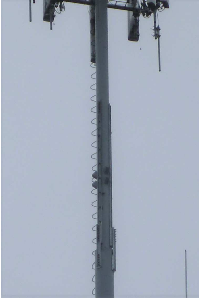
Photo 2: Reinforcement Channel w/Bridge Stiffeners from approximately 121' to 136'
