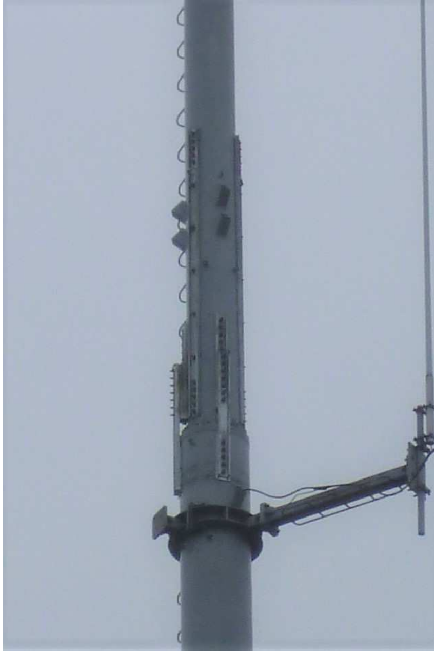
Photo 3: Reinforcement Channel w/Bridge Stiffeners from approximately 99' to 111'
