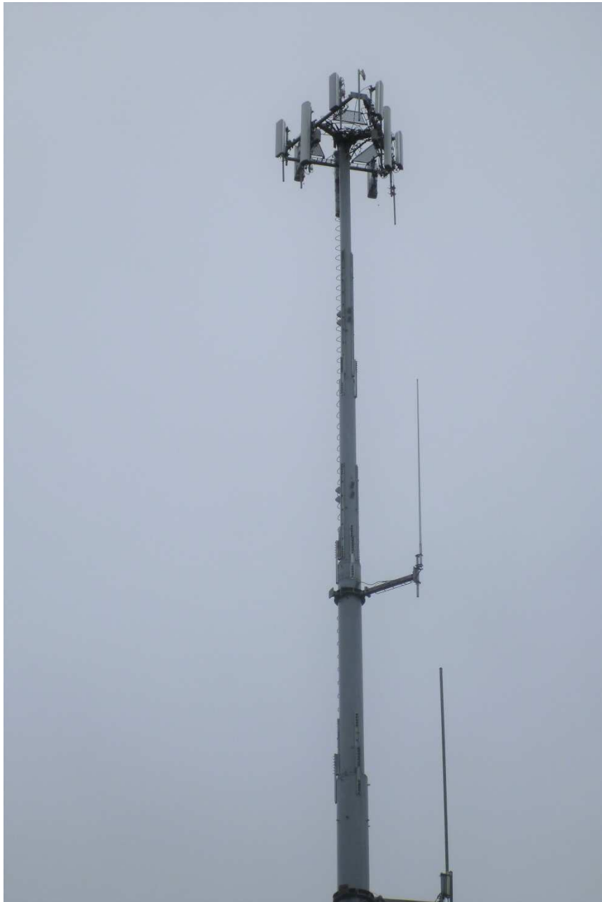
Photo 1: Partial Monopole Elevation
