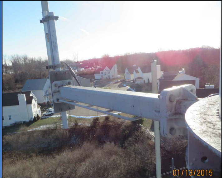
Photo From Tower
