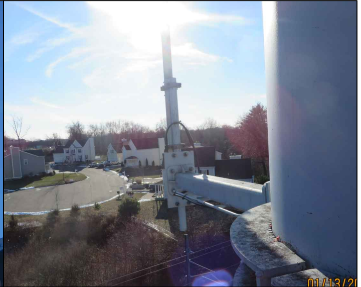
Photo From Tower
