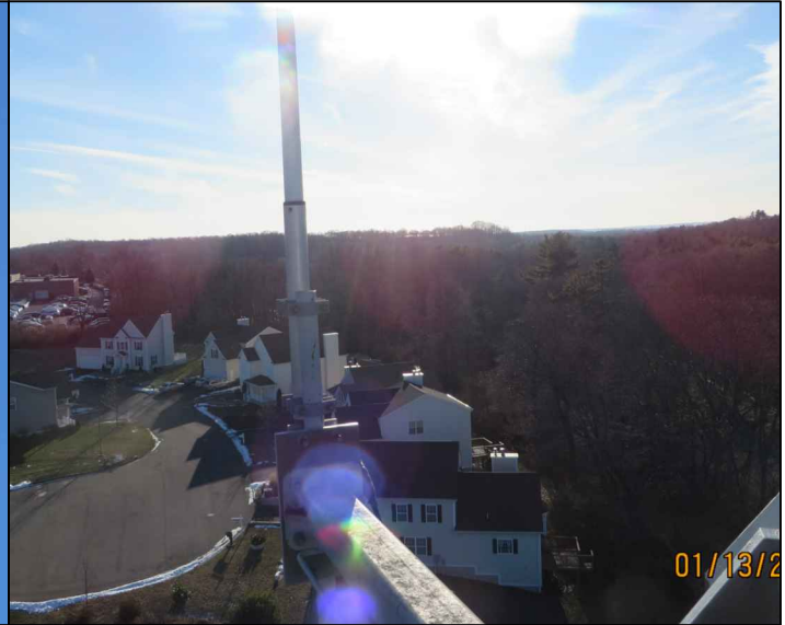
Photo From Tower
