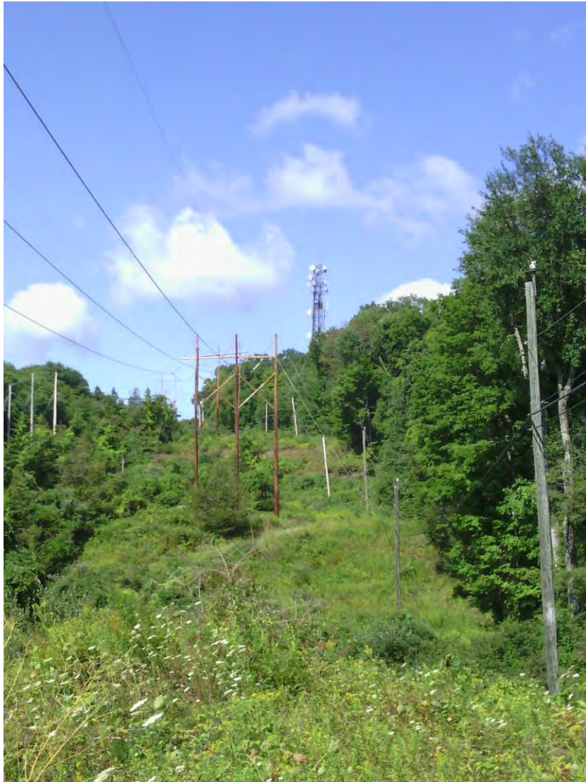
Existing tower from CL&P right-of-way, view west.
