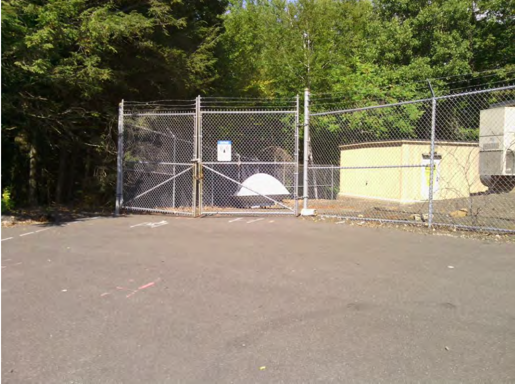
South side of compound - proposed tower location by white dome. Compound would be expanded to the left (west).
