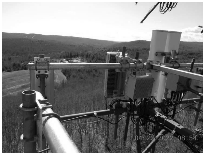
Fig. 1: Overall View of Antennas, RRHs & OVP in Alpha Sector
