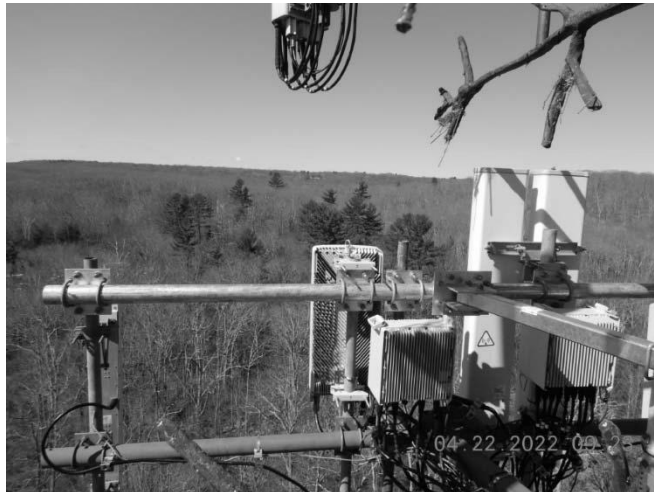
Fig. 2: Overall View of Antennas, RRHs & OVP in Beta Sector
