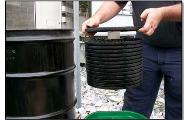
Note: OLTC Filter Maintenance
