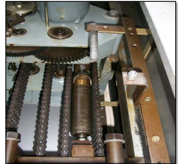
Note: Breaker inspection & repairs
