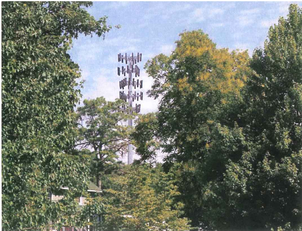
Branford Site photo-simulation 2 - Adjacent to #180 Short Beach Road, 0.09 miles south.
