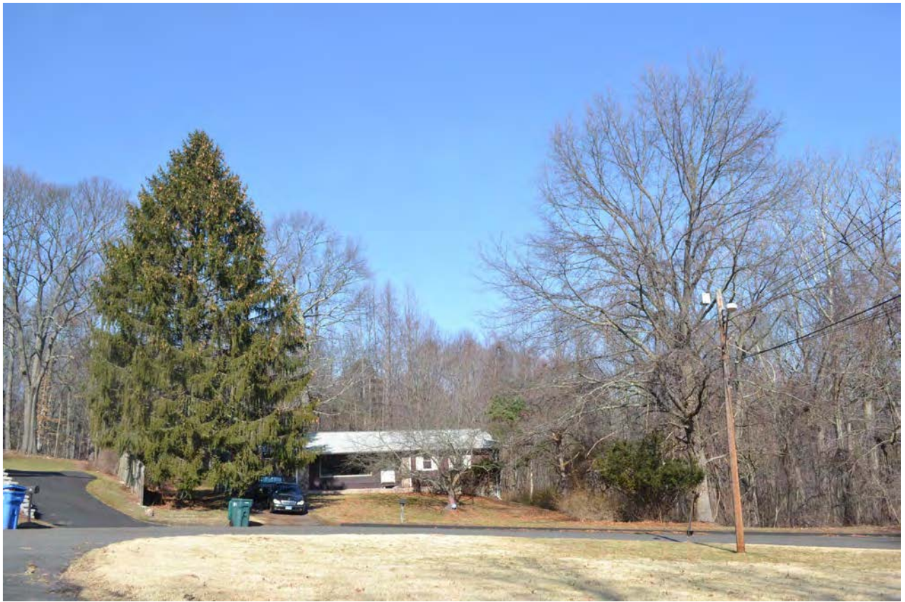
Photograph 19. View looking northeast towards the Subject Property from Tierney Road. 2/21/2018.
