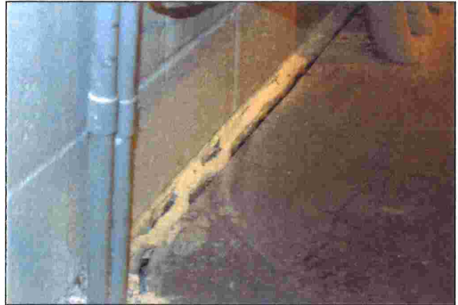
Figure 10: Building Wall Separation
