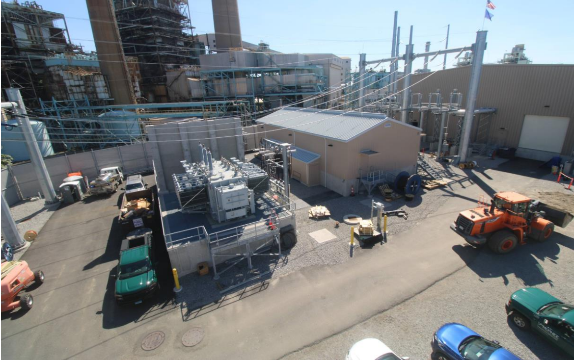
Photo 1: Broadview of project site with GIS/Control and PDC building exteriors completed.
