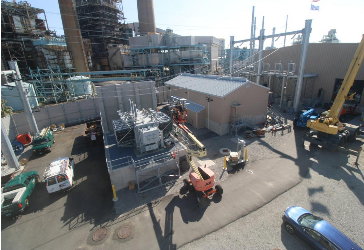
Photo 1: Broadview of project site with GIS/Control and PDC building exteriors completed.
