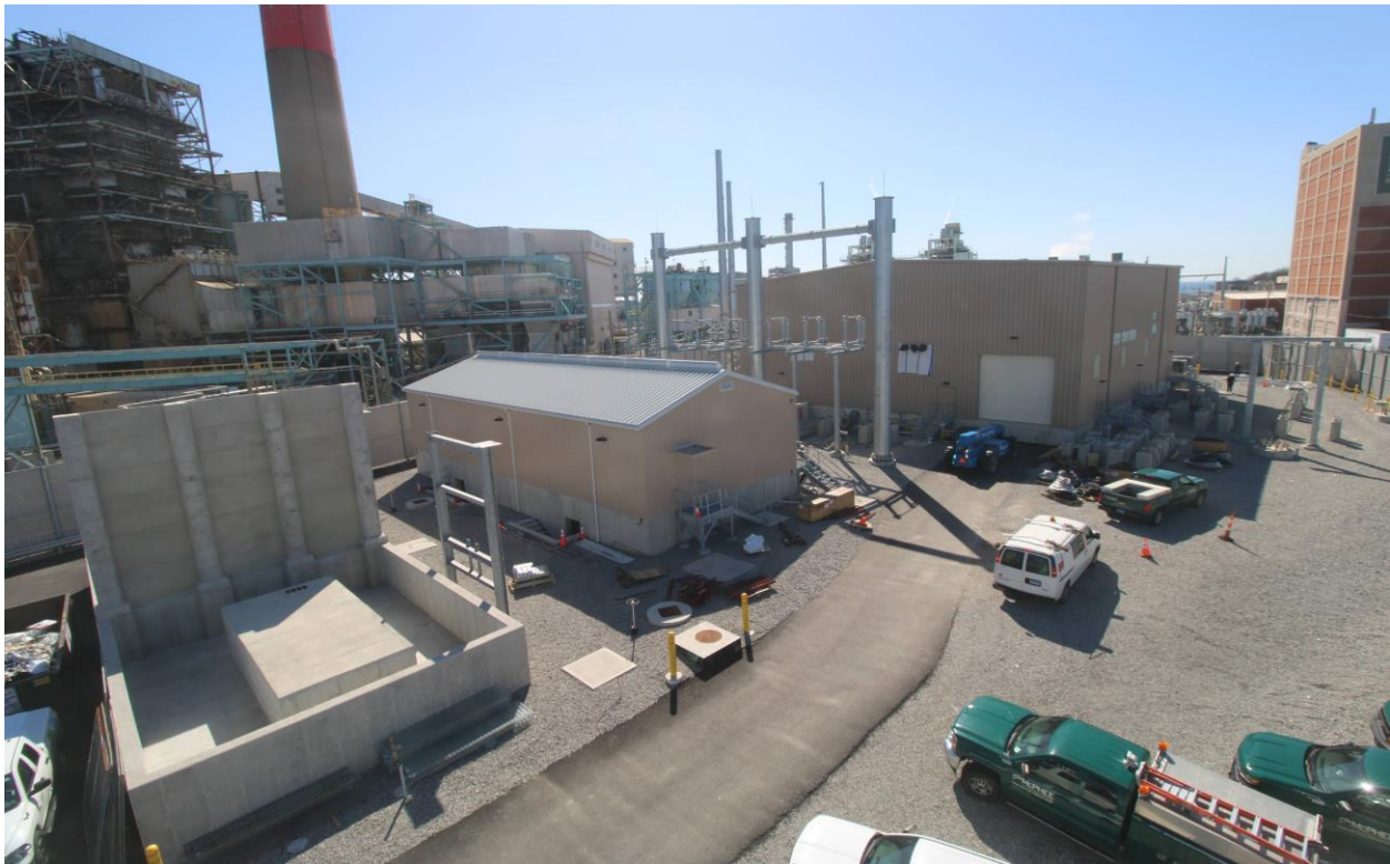
Photo 1: Broadview of project site with GIS/Control and PDC building exteriors completed.
