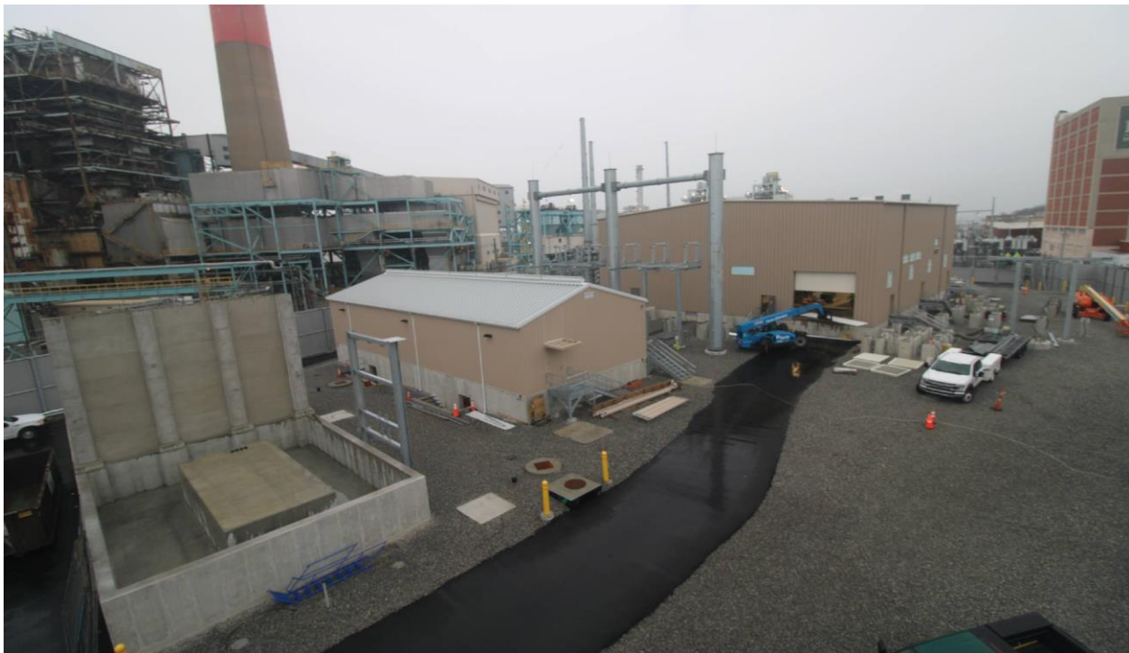
Photo 1: Broadview of project site with GIS/Control and PDC building exteriors completed.
