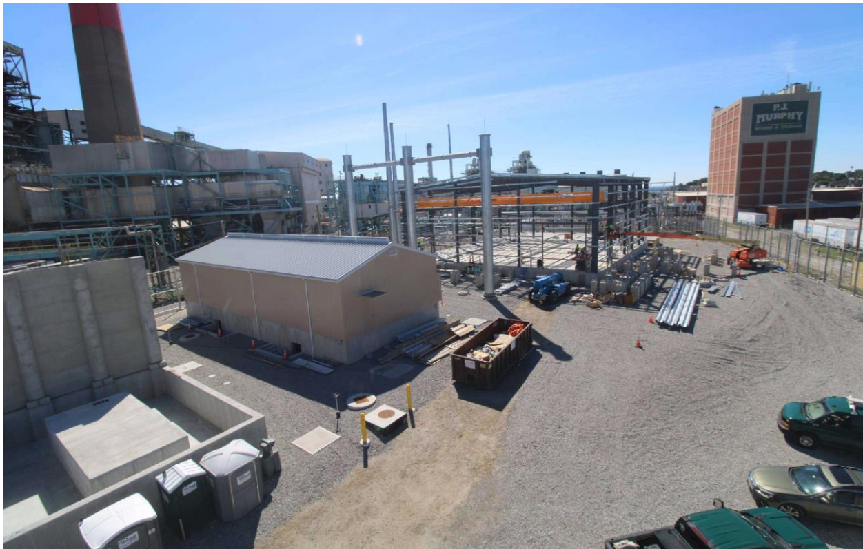
Photo 1: Broadview of project site with GIS/Control Building being erected.
