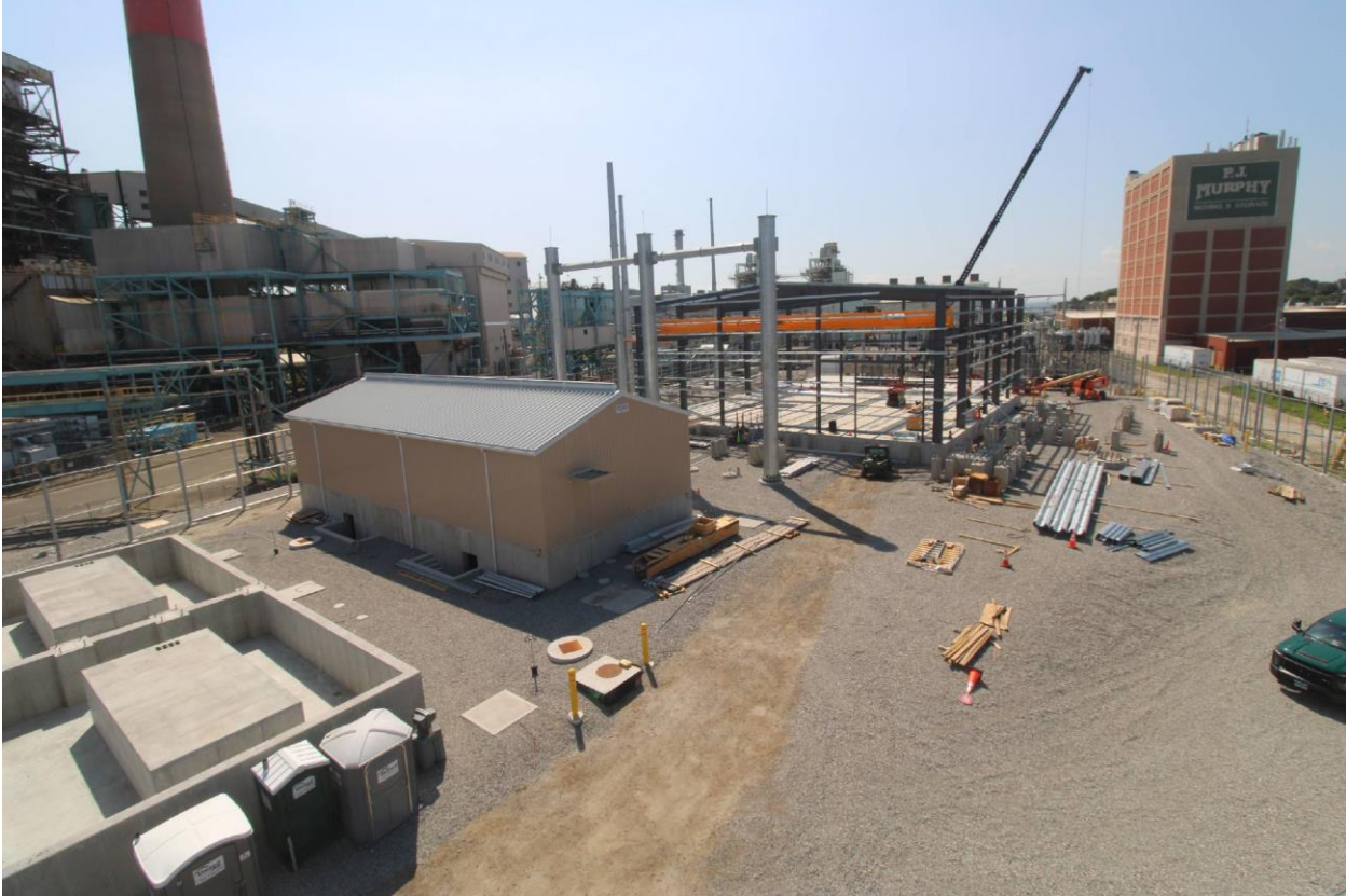
Photo 1: Broadview of project site with GIS/Control Building being erected.
