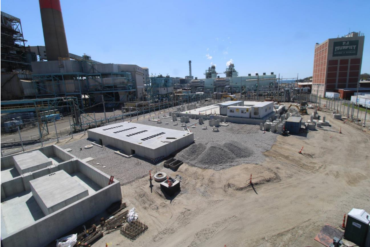
Photo 1: Broadview of project site with TXF and GIS foundation walls installed.
