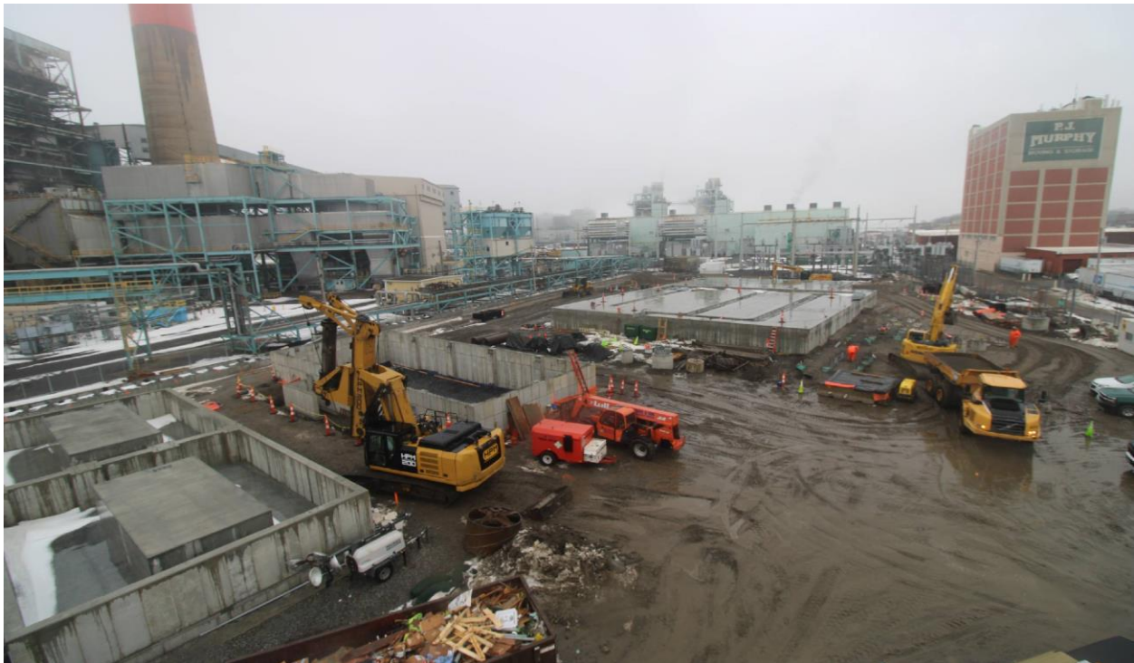
Photo 1: Broadview of project site with TXF and GIS foundation walls being installed.
