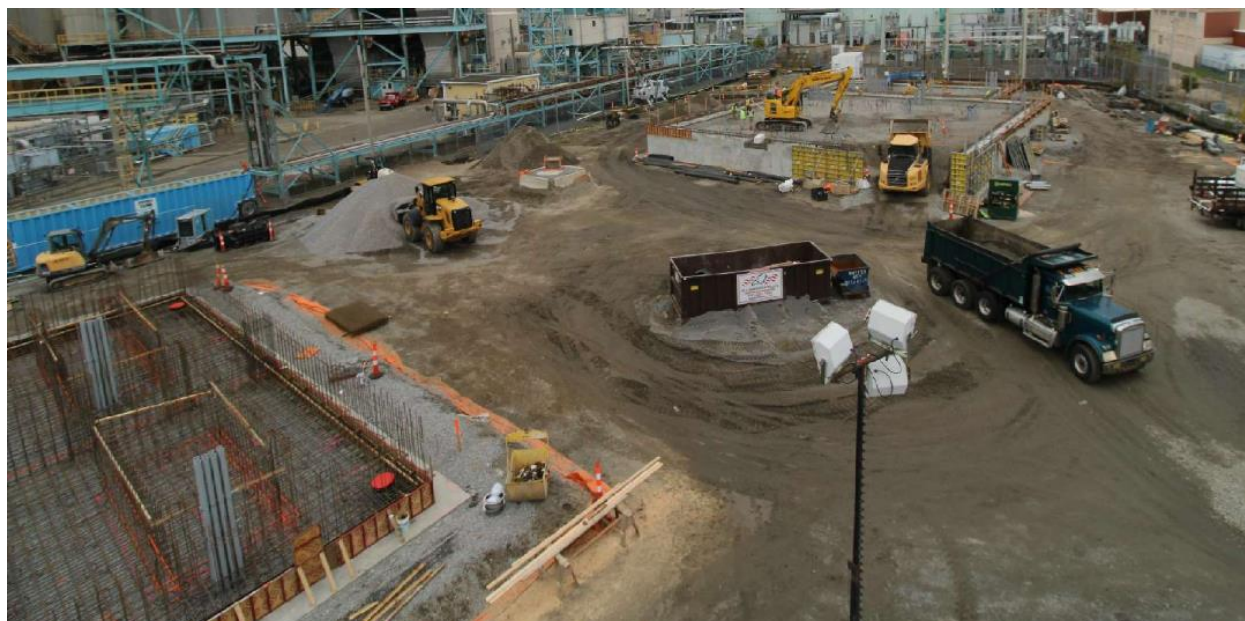
Photo 1: Broadview of project site with foundation walls being installed.
