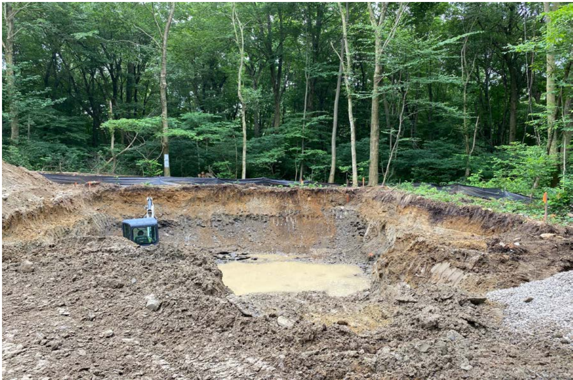
Photo 4: View of tower foundation excavation work underway looking east.
