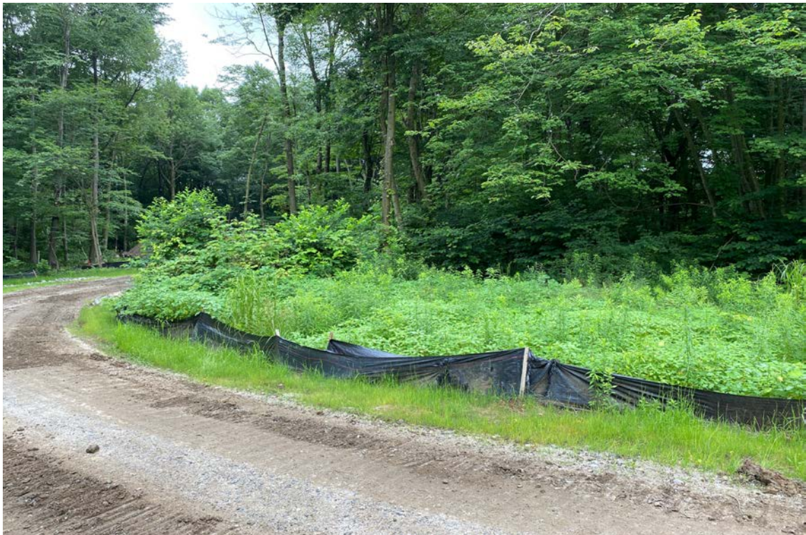
Photo 8: View of erosion controls in proximity to Wetland 1 looking south; all controls found in good condition.
