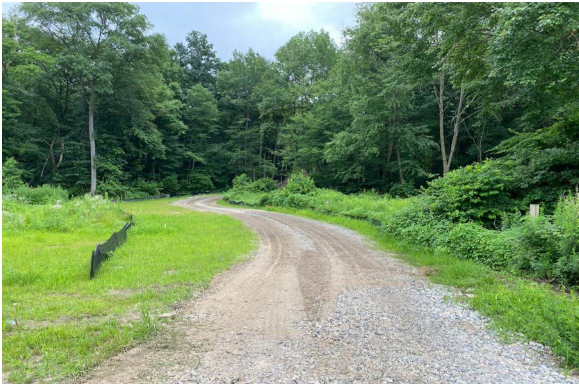
Photo 2: View of access road looking south showing shoulder stabilized with well established permanent vegetation.
