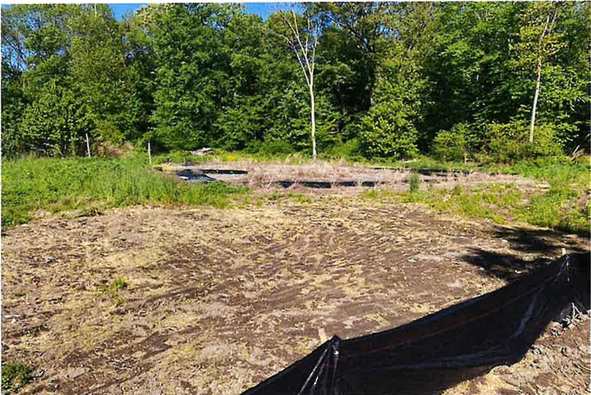
Photo 6: View of removed temporary stockpile area seeded and mulched; seed mix just starting to germinate.
