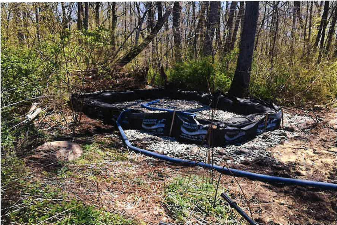
Photo 2: View of temporary dewatering basin for access road construction looking southeast.
