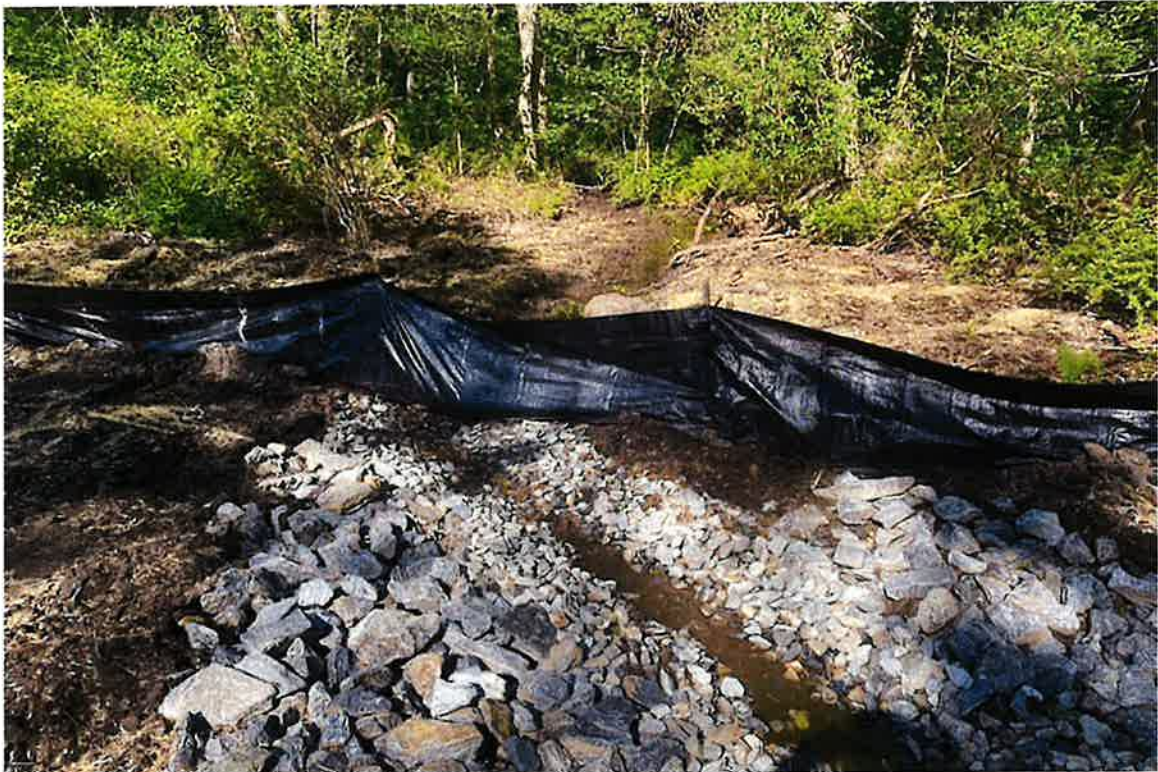
Photo 4: View of southern culvert outlet looking east.
