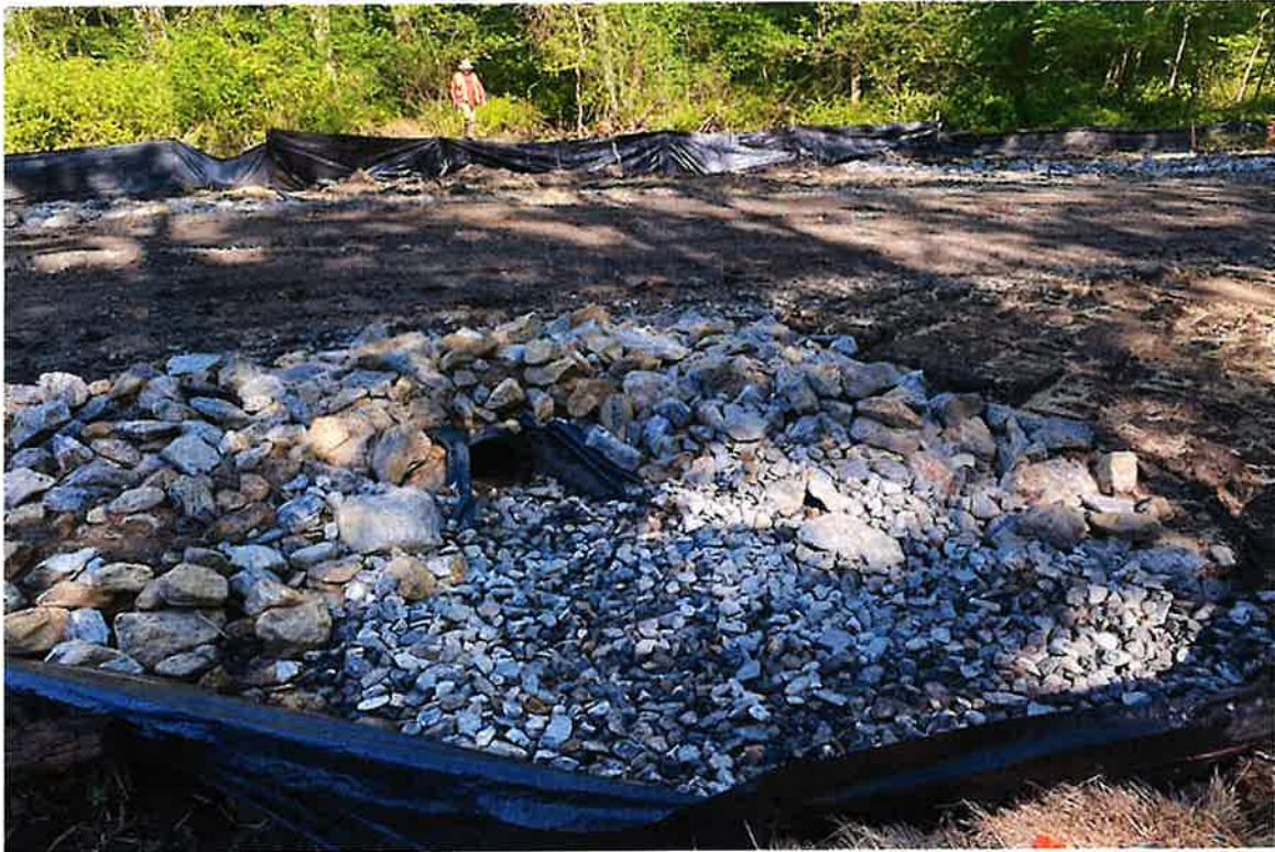
Photo 3: View of northern culvert inlet looking east.
