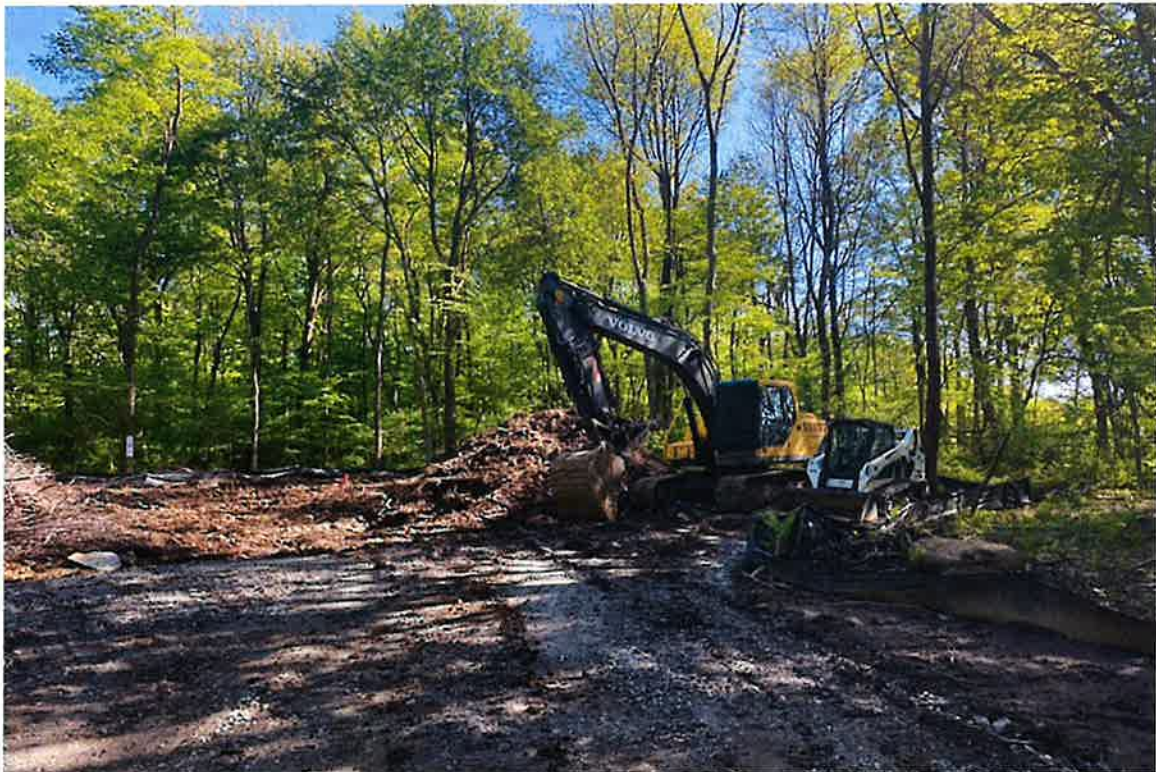
Photo 8: View of cleared tower compound area looking south.
