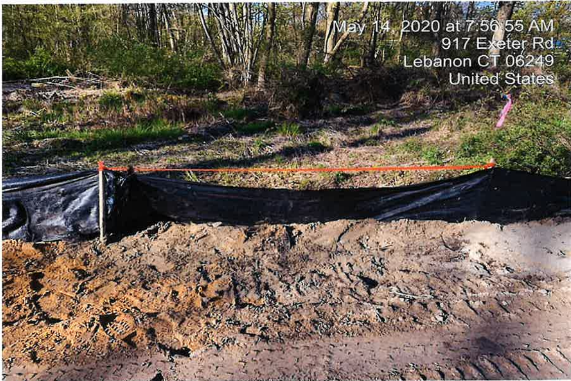
Photo 5: View of repaired silt fence.
