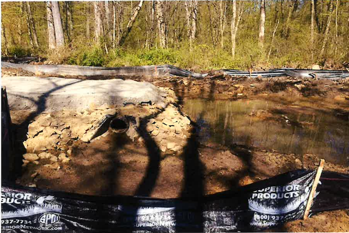
Photo 3: View of culvert and French mattress.
