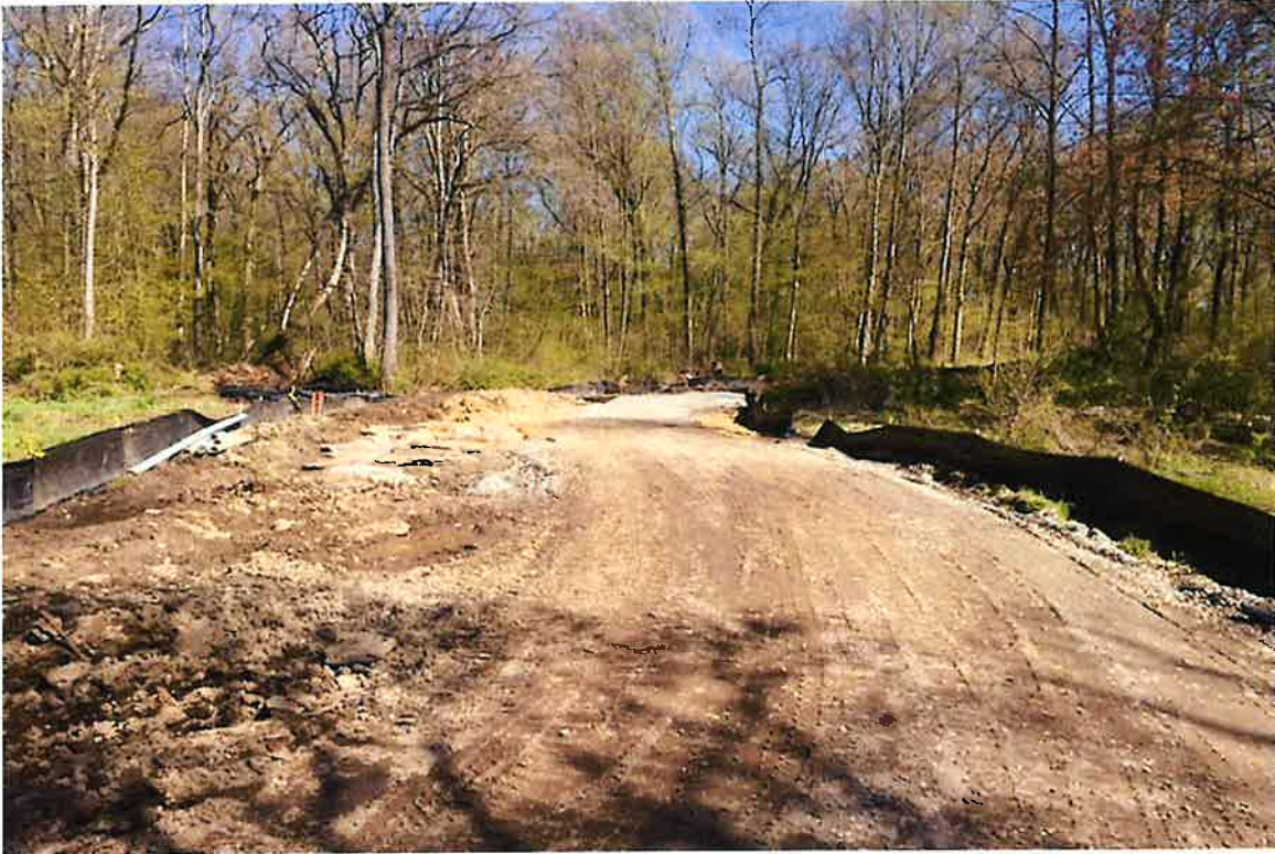
Photo 1: View of access road under construction looking south.
