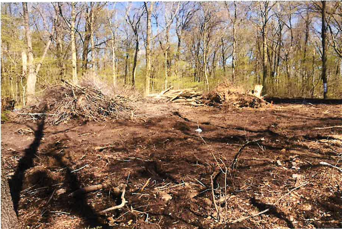
Photo 2: View of compound looking south.
