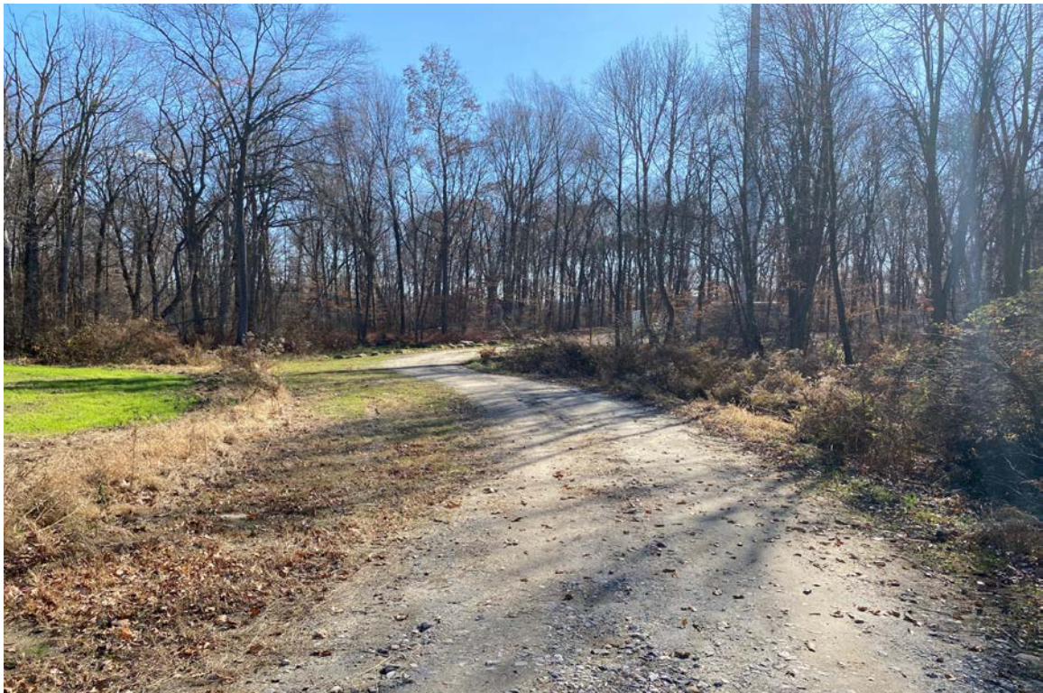
Photo 2: View of access road looking south showing shoulder stabilized with well established permanent vegetation and erosion controls removed.
