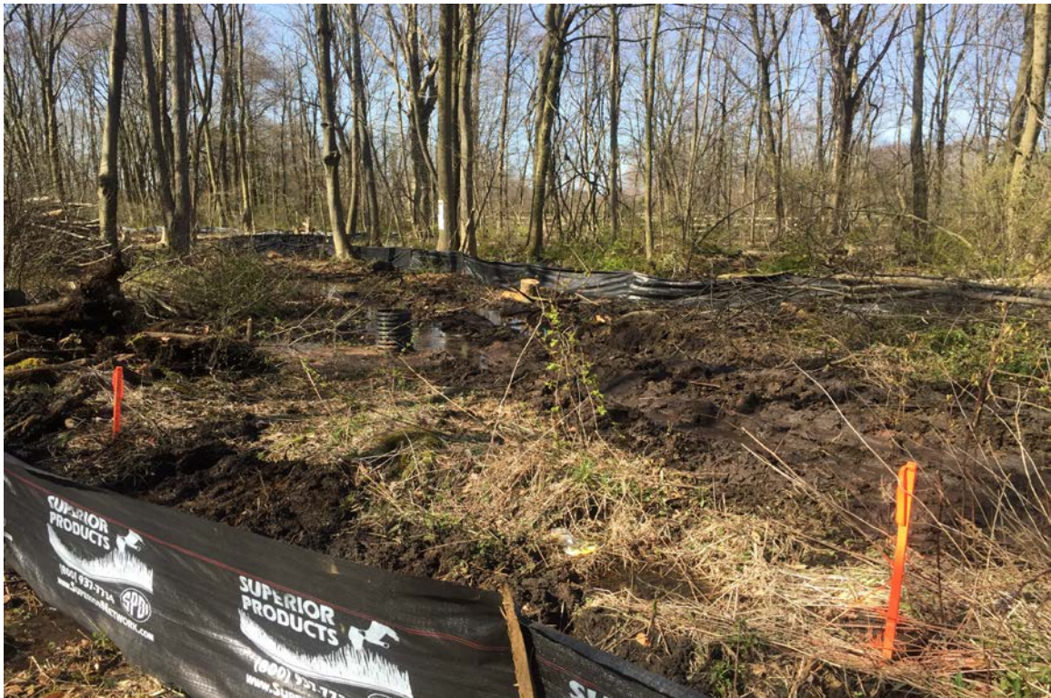
Photo 2: View of proposed culvert and French mattress location looking west. Orange survey stake in left side of photo depicts the location of STA 2+64.46.
