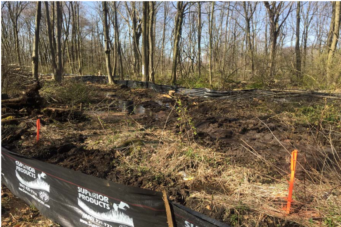
Photo 2: View of proposed culvert and French mattress location looking west. Orange survey stake in left side of photo depicts the location of STA 2+64.46.
