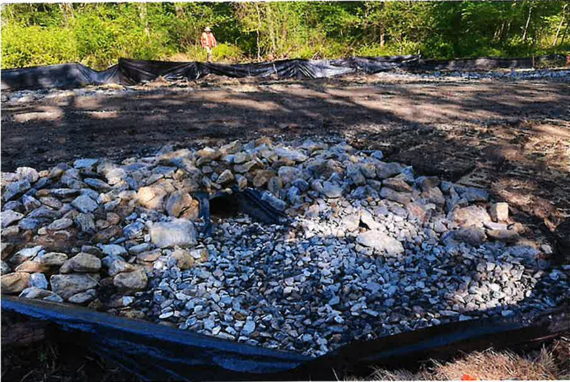
Photo 3: View of northern culvert inlet looking east.
