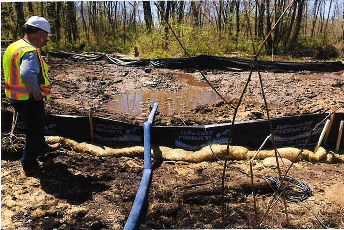
Photo 3: View of the dewatering access road looking west.
