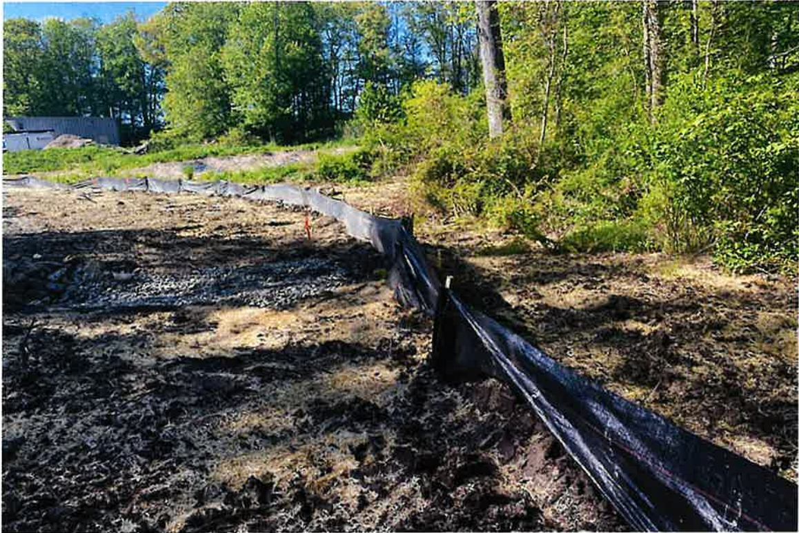
Photo 7: Typical view of silt fence; all found in good condition.
