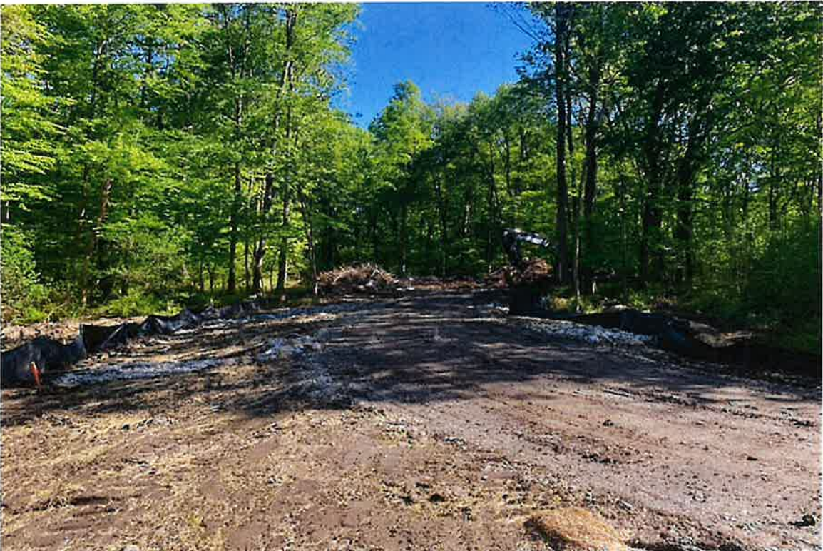
Photo 2: View of access road looking south across French mattress and two culverts section of road with compound in background.
