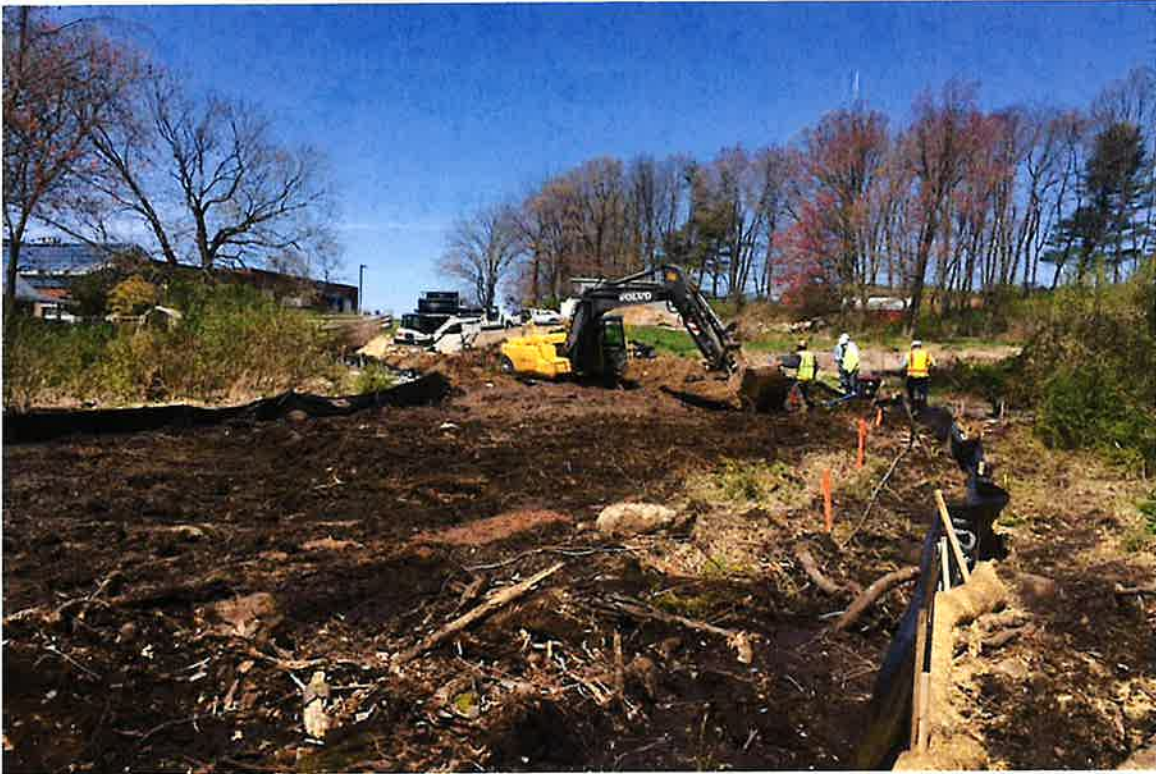
Photo 1: View of access road under construction looking north.
