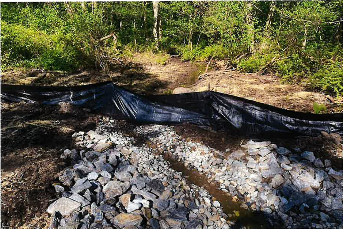
Photo 4: View of southern culvert outlet looking east.
