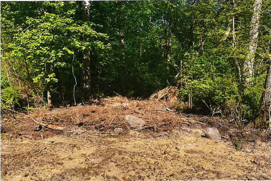
Photo 5: View of removed temp dewatering basin area seeded and mulched; seed mix just starting to germinate.
