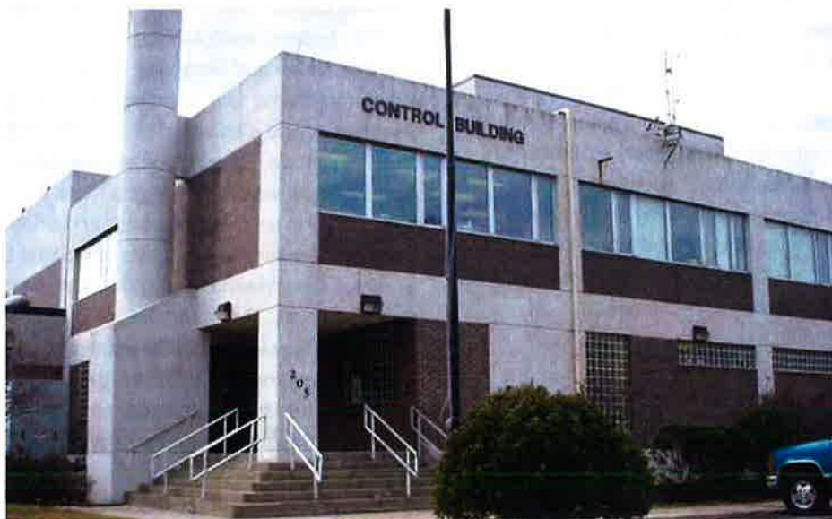
WPCA Treatment Plant | Source: City of Bridgeport
