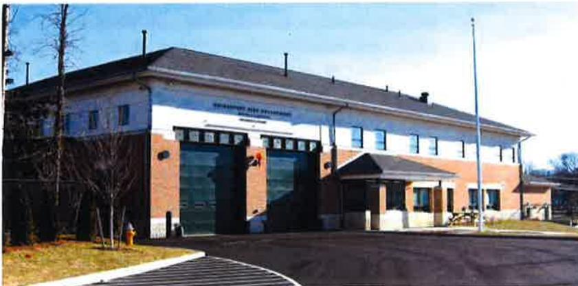
Newly constructed firehouse on Boston Avenue | Source: City of Bridgeport Fire Department
