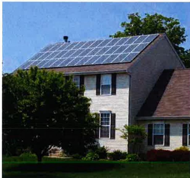
Roof-mounted solar panels | Source: Stantec
