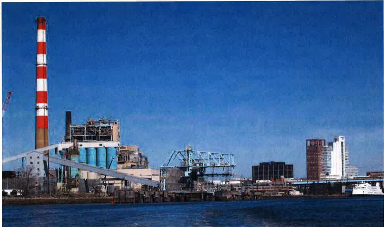
Power generation in the South End | Source: Stantec
