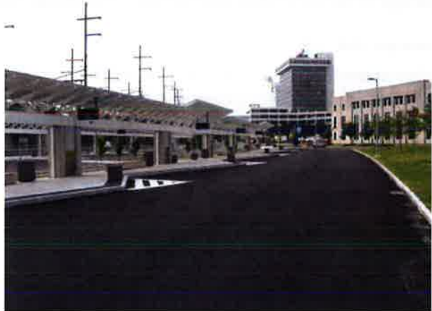
Inter-modal Center (front view) | Source: Stantec
