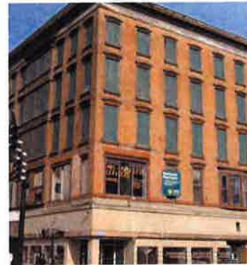
Part of the Downtown North Historic Rehabilitation project | Source: Phillips Preiss Shapiro Associates
