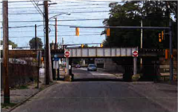
New Haven Rail Line | Source: Stantec
