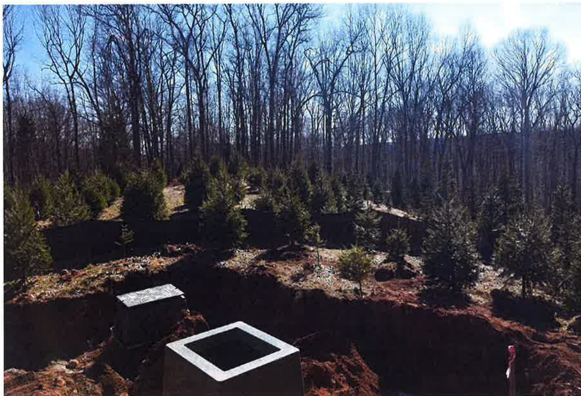
Photo 6: View of ongoing utility trenching work.
