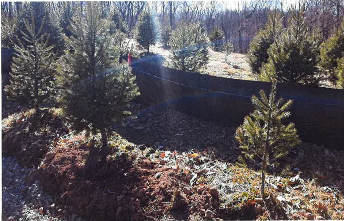
Photo 5: View of exclusionary silt fence properly installed.
