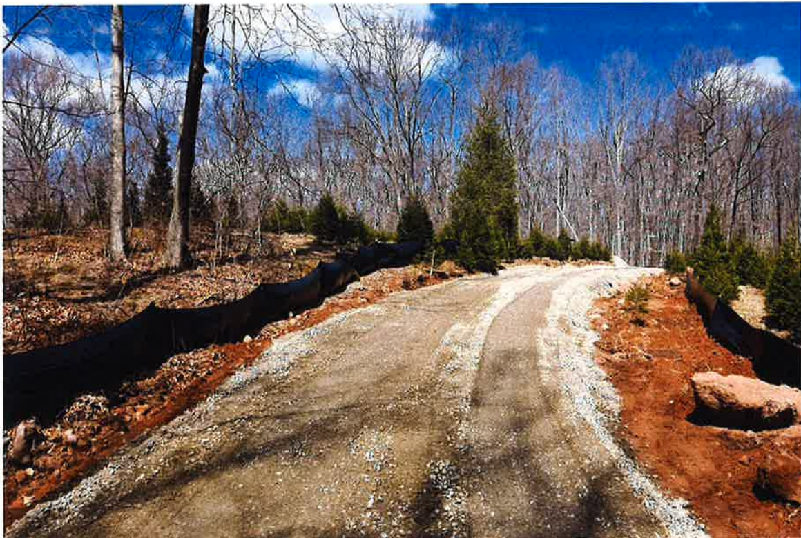
Photo 4: View of completed gravel access road.
