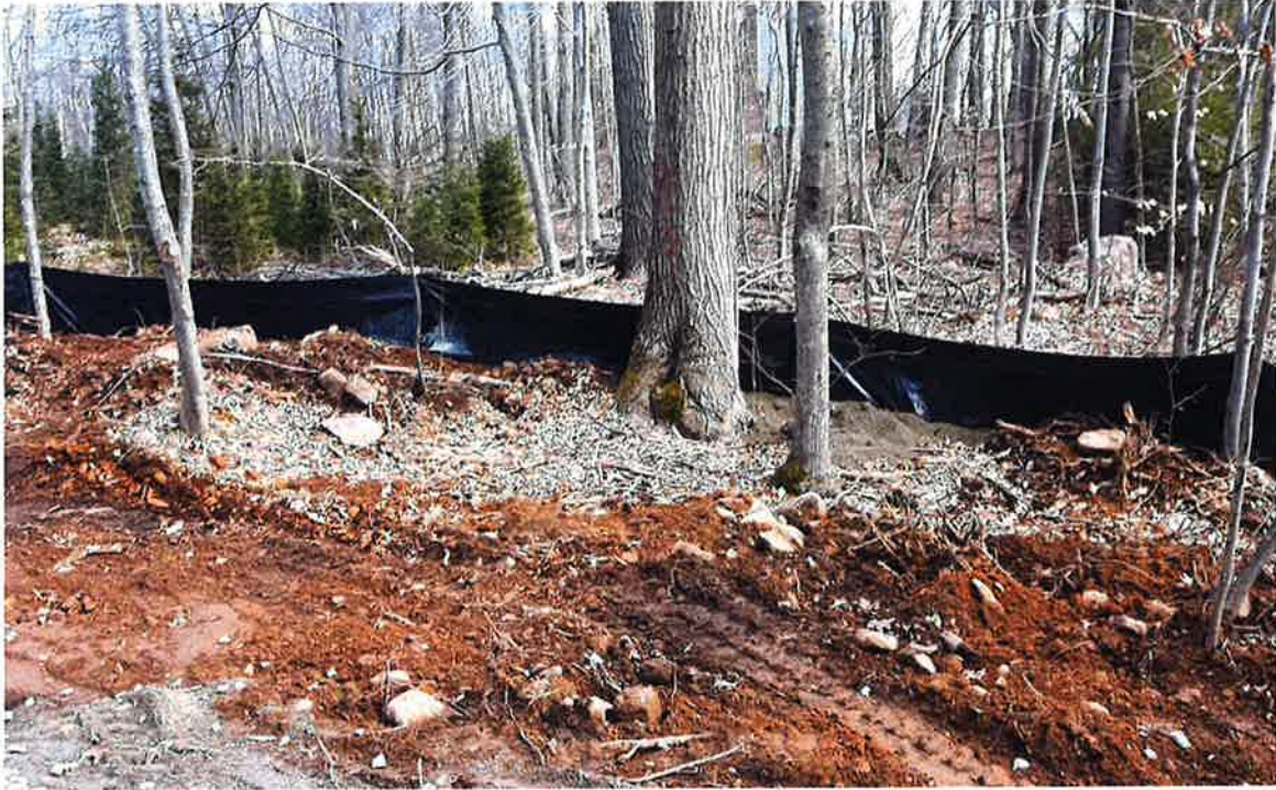
Photo 3: View of properly installed exclusionary silt fence.
