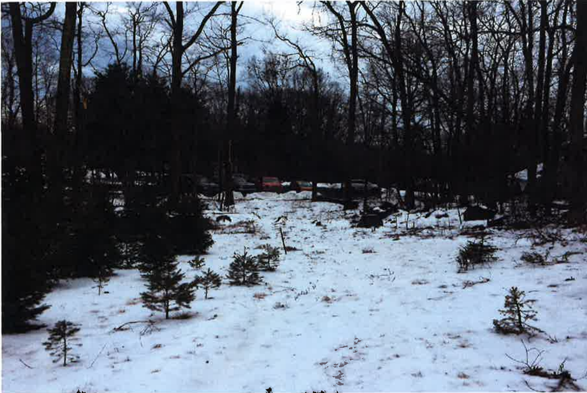
Photo 1: View of construction access entrance prior to work start.
