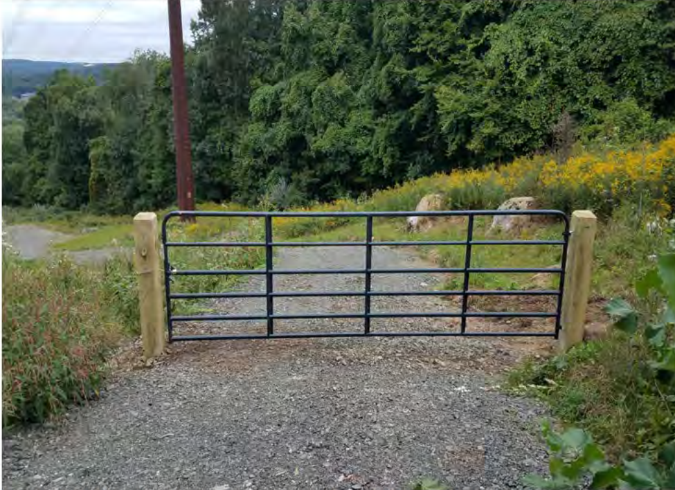
Photo 9: 09/20/2018, Bethel: Map 07, view of access road to Str1014 and installed security gate. Final grading (pad and access road) and initial restoration has been performed. Photo taken facing west from Hearthstone Drive towards Str1014 in the distance.
