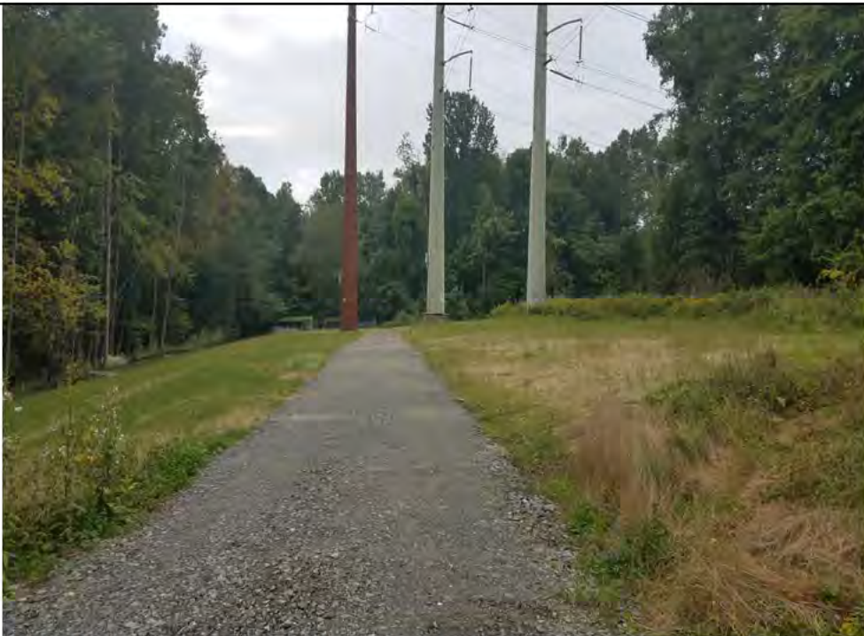
Photo 10: 09/20/2018, Bethel: Map 07-08, view of Structure Str1015 (Map 07) and the permanent access road off of Chimney Drive (Map 08). Final pad and access road grading, and initial restoration has been performed. Photo taken facing south from Chimney Drive towards Str1015 in the distance.
