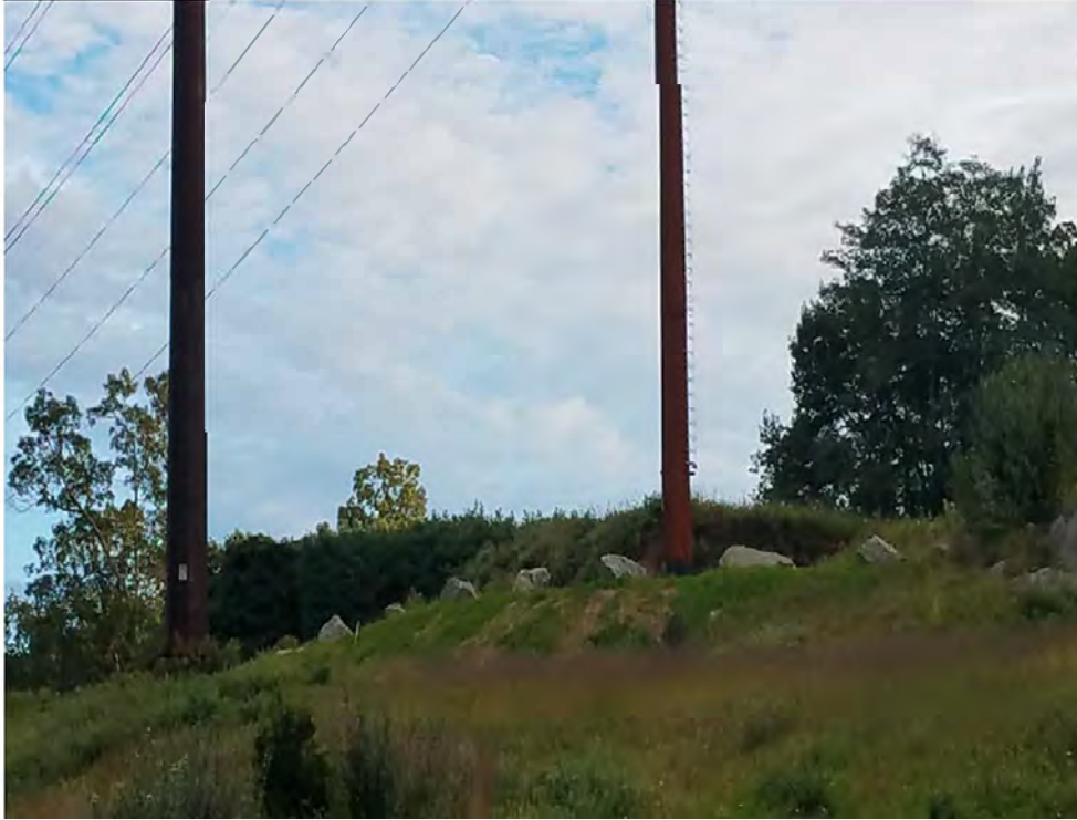
Photo 15: 09/27/2018, Bethel/Brookfield: Map 12, Str1023, view of west slope of work pad where previous erosion occurred. Area has been stabilized with seed and straw mulch. At the time of this inspection grass was growing and no erosion was observed.
